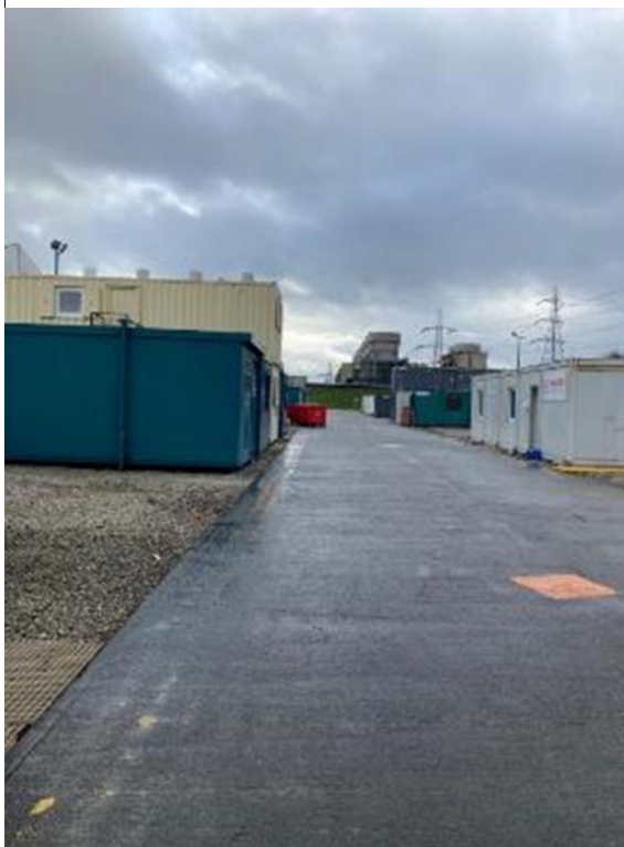
Building 4 - Negligible bat roost suitability
