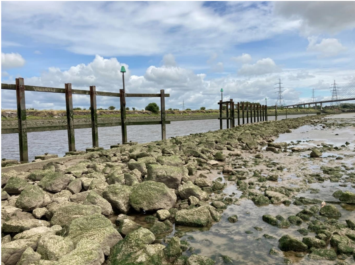
Plate A-13: Boulders placed around outfall infrastructure
