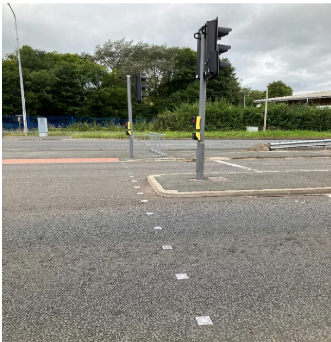
Figure 3.6 | Controlled crossing/Junction, Orion Service
