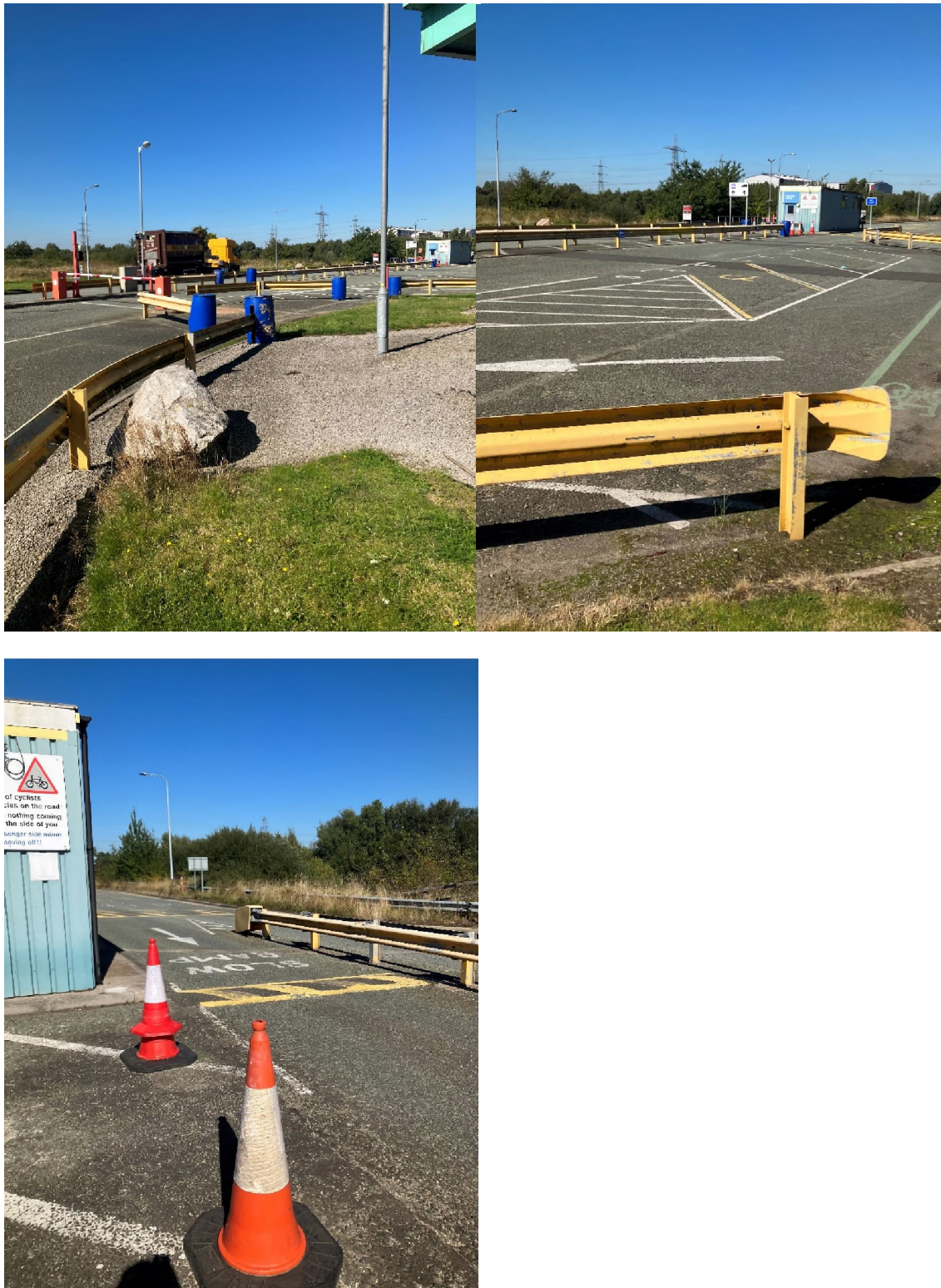
Figure 4.6 | Tata Steel Gate House Exit Lane
