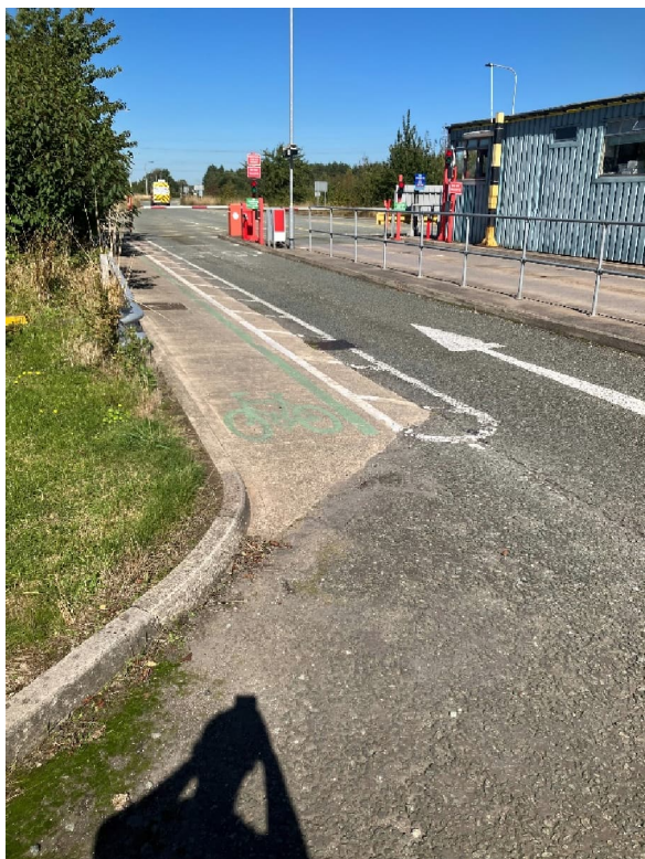
Figure 4.5 | Tata Steel Gate House Exit Lane
