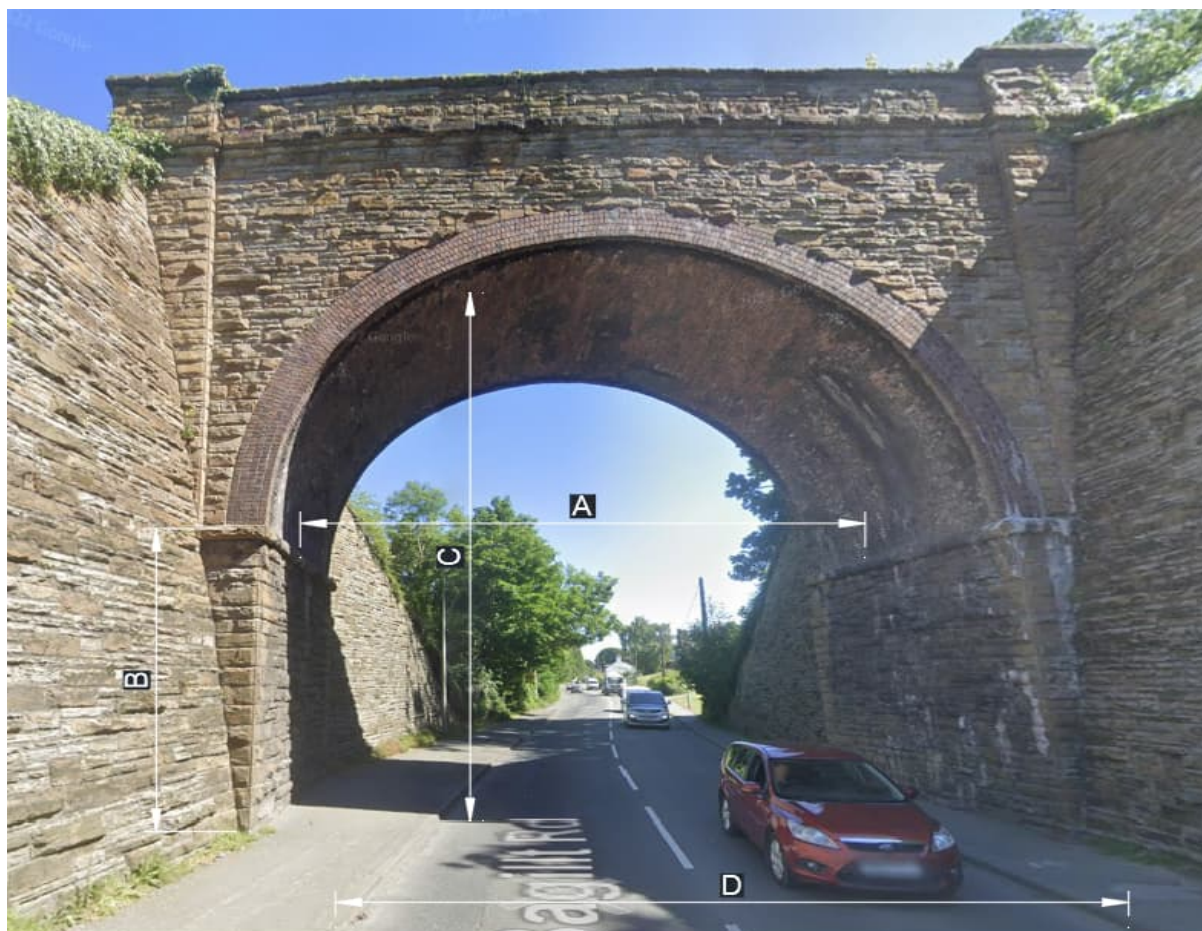
Figure 3.5 | Grade II overbridge
