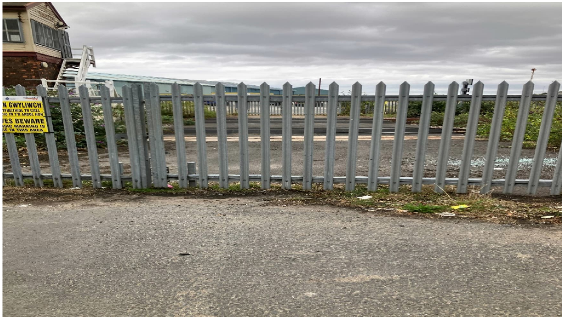
Figure 3.2 | Mostyn point, Site Gate at Egress Location onto A548
