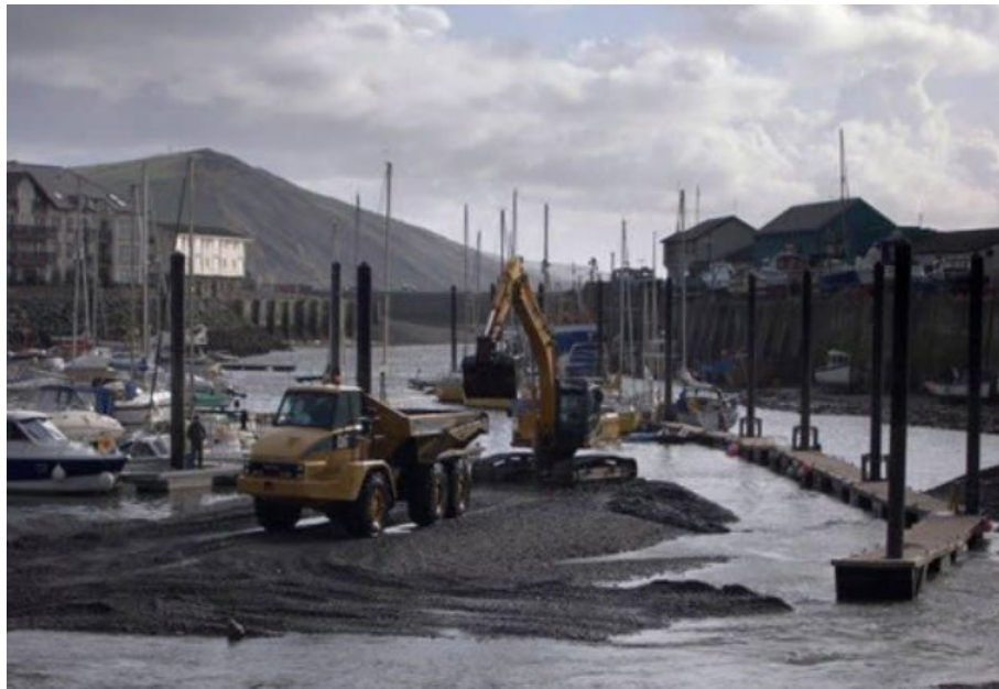
Figure 3 Dredging of the harbour in 2008
