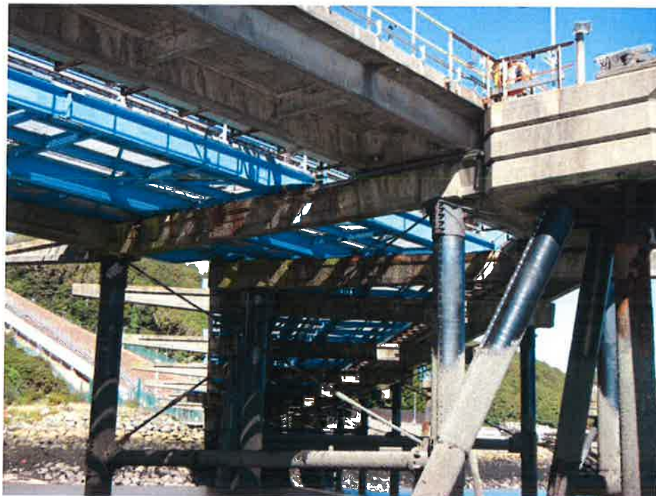
Figure 9: EMD6 - Prepare, inspect and paint central pile and bracing/clamp
