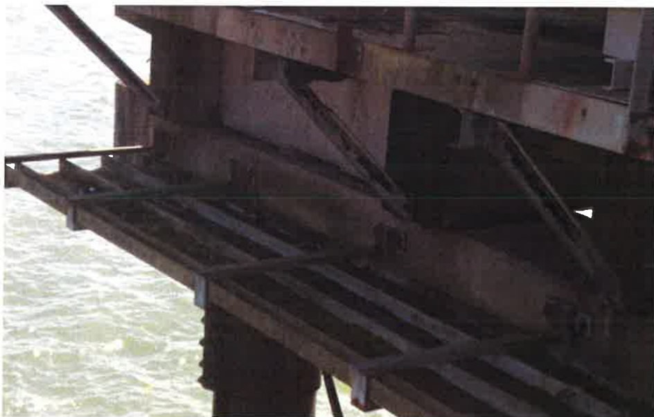
Figure 5: Support bracing - Prepare, inspect and paint bracing/support
