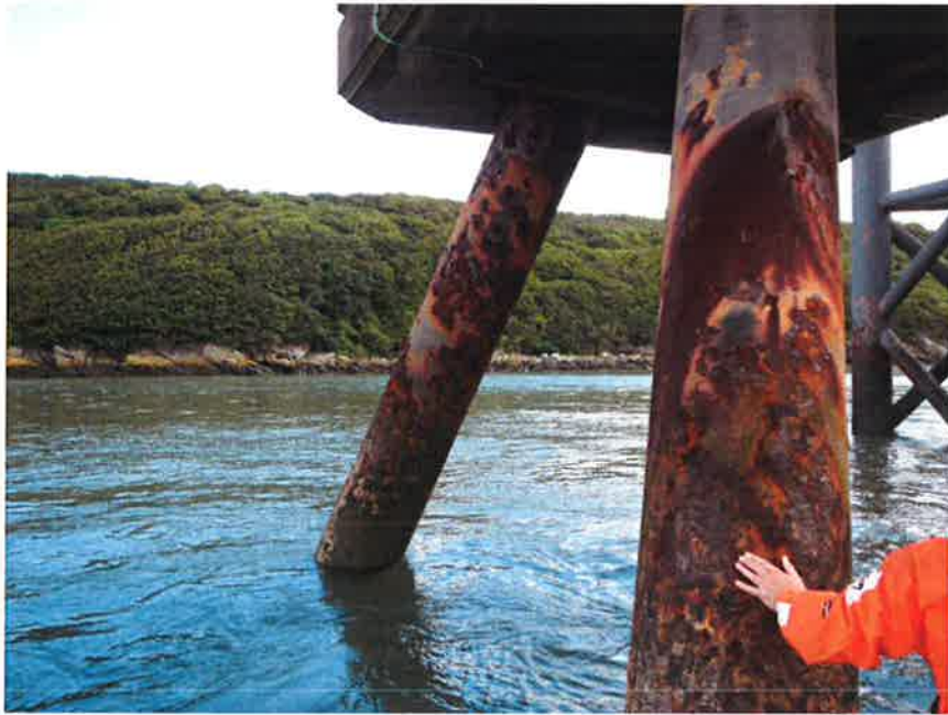
Figure 2: EMD3 - Prepare, inspect and paint 5 off piles
