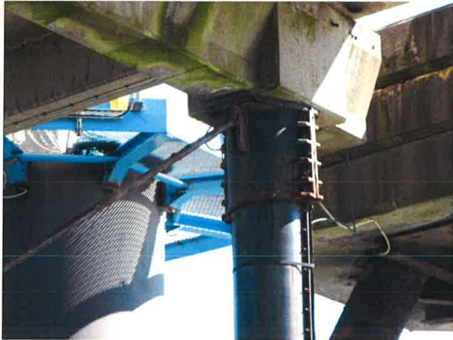
Figure 6: EMD4 - Cross bracing
