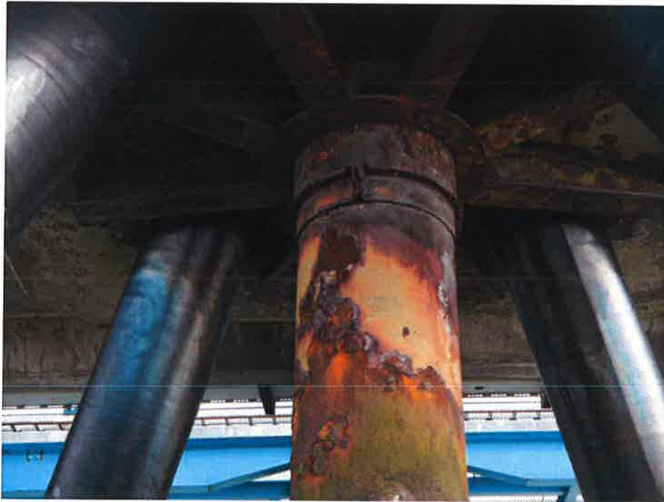
Figure 8: EMD6 underside - Prepare, inspect and paint central pile
