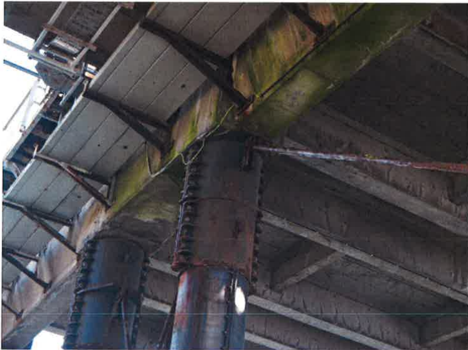
Figure 4: Cross bracing at Jetty head - Prepare, inspect and paint bracing and clamps
