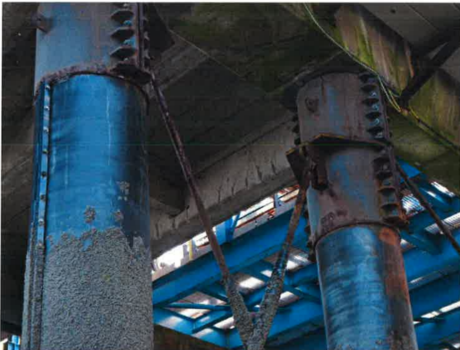
Figure 3: Cross bracing at Jetty head - Prepare, inspect and paint bracing and clamps
