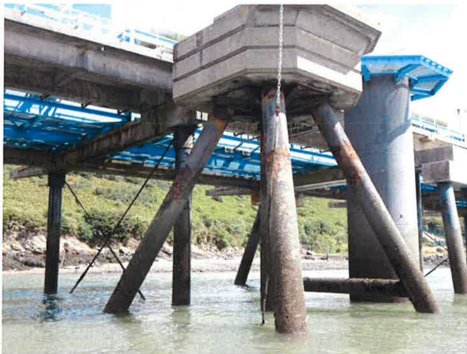
Figure 7: EMD4 - Prepare, inspect and paint 5 off piles, bracing and clamp
