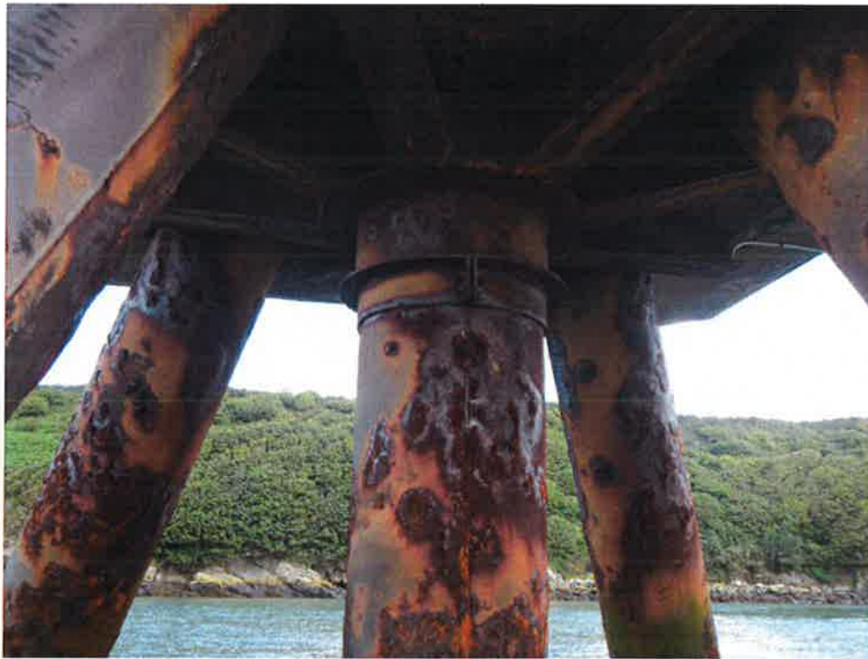
Figure 1: EMD3 - Prepare, inspect and paint 5 off piles
