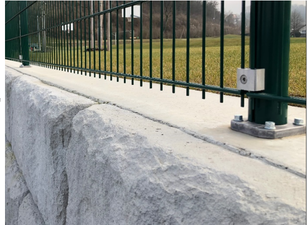
Photograph 1 - example of fence posts fitted to Redi-rock blocks
