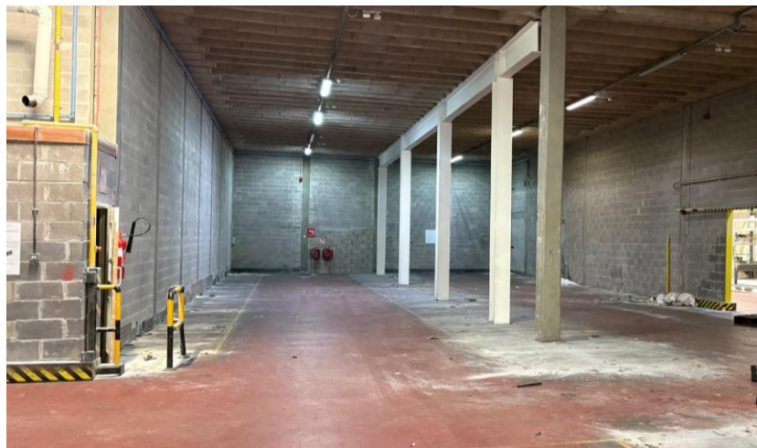
Figure 14: Blending Plant – Middle Floor
