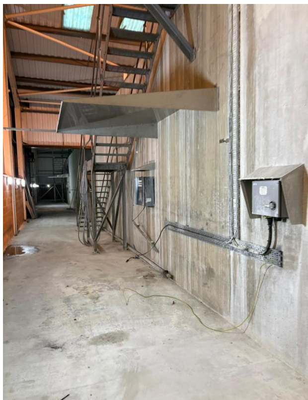
Figure 4: New Farm Blower Area
