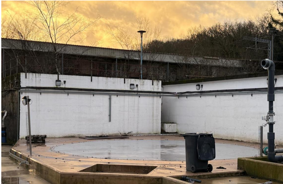
Figure 16: A21 Balance Tank Removed
