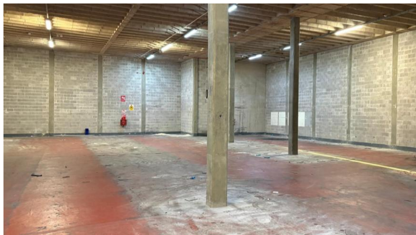
Figure 15: Blending Plant – Top Floor
