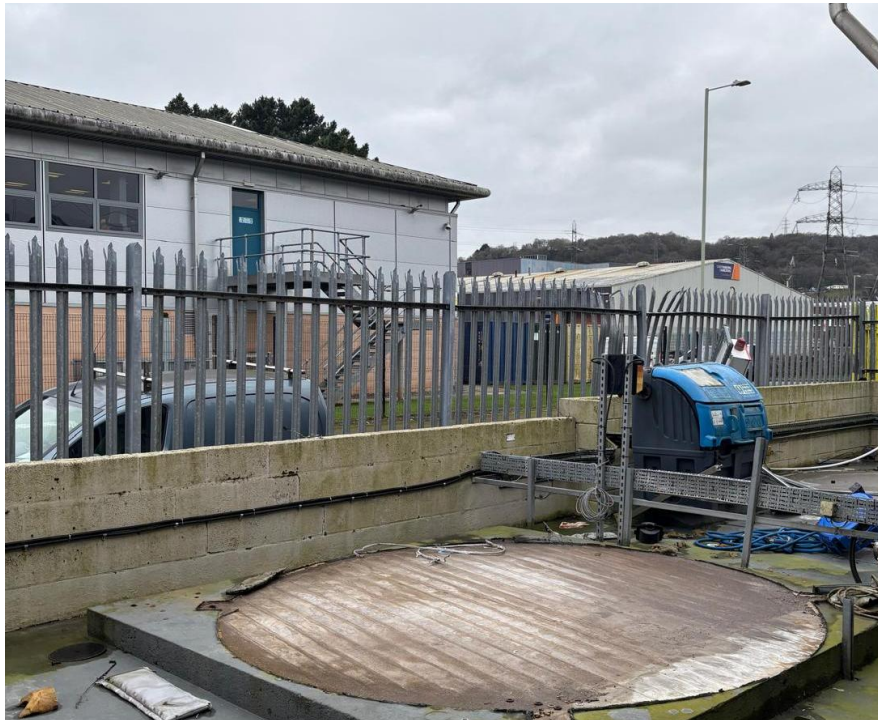
Figure 7: Removed Water Tank
