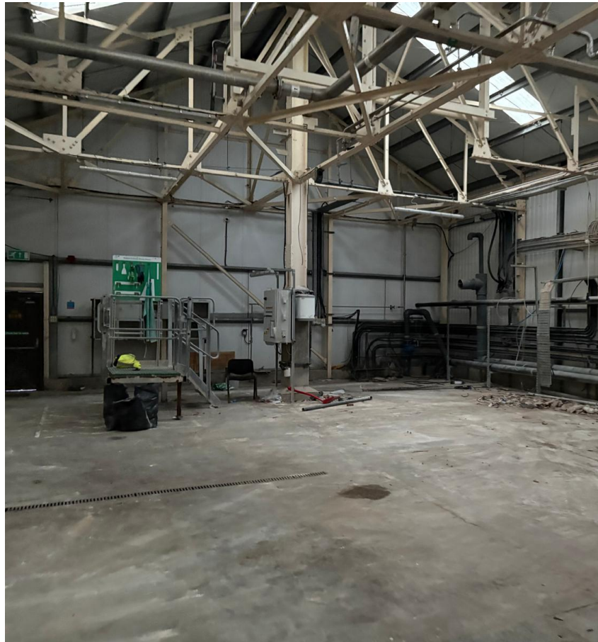
Figure 9: A18 Effluent Plant – DAF Area
