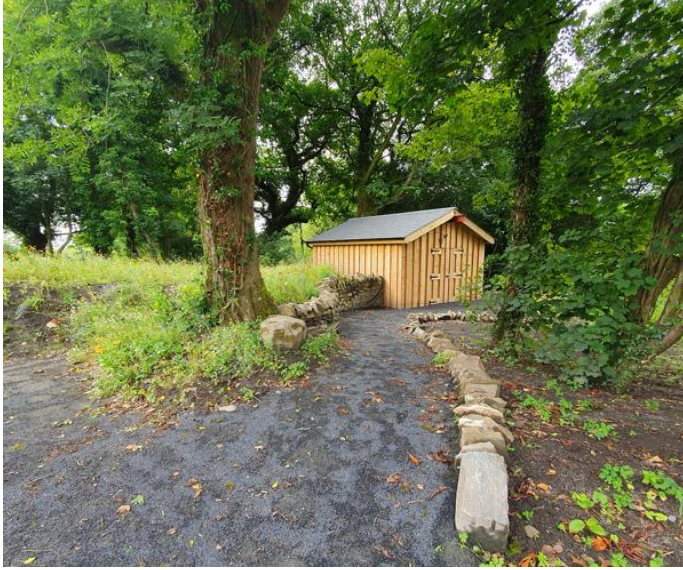
Powerhouse Location (existing)
