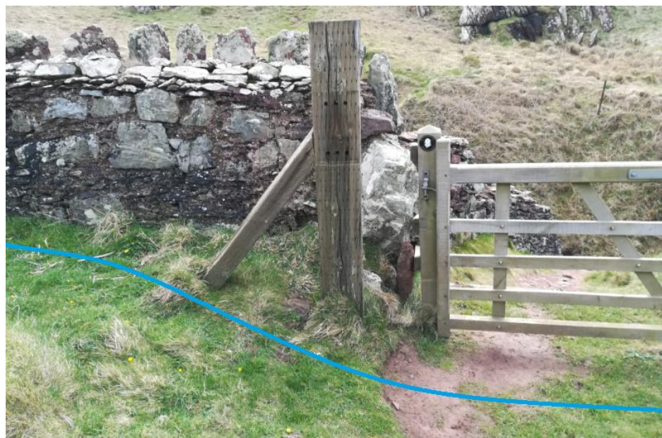
Figure 2.12 Recently installed footpath gate and cable crossing point.
