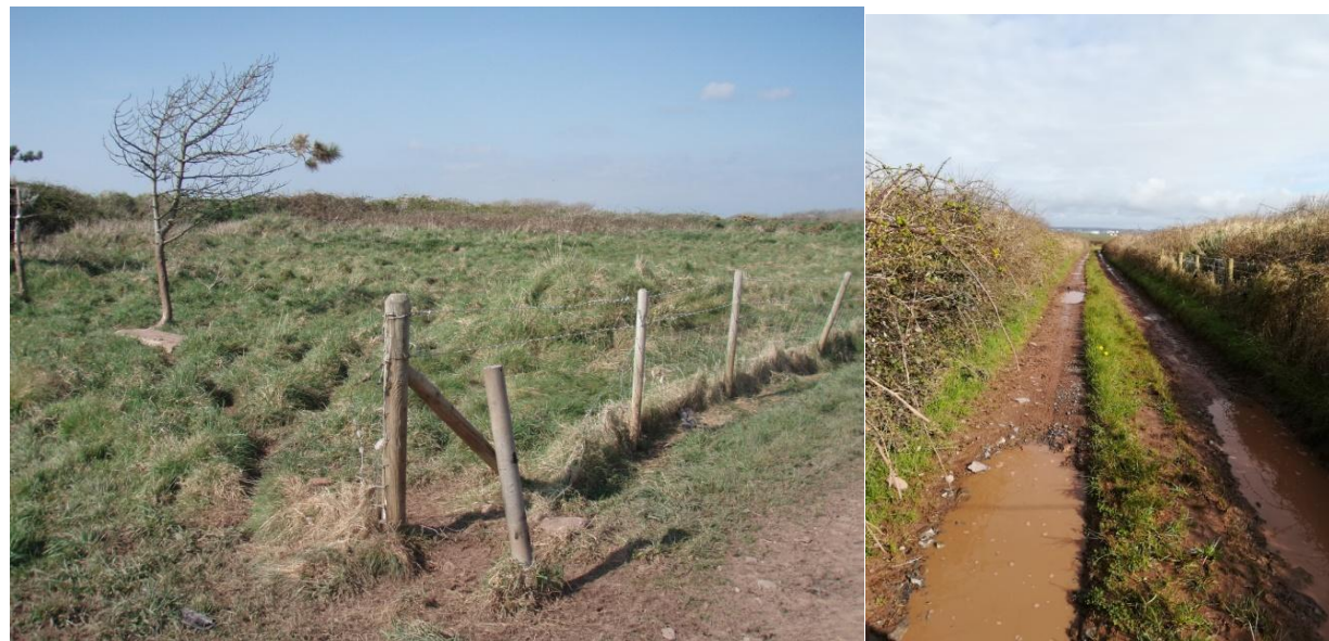
Figure 2.14a showing control station site and 2.14b access track from main road
