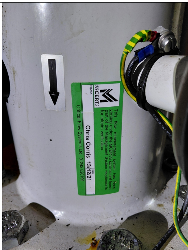
Photograph 2: Magflow meter at the abstraction point within 5 year calibration
