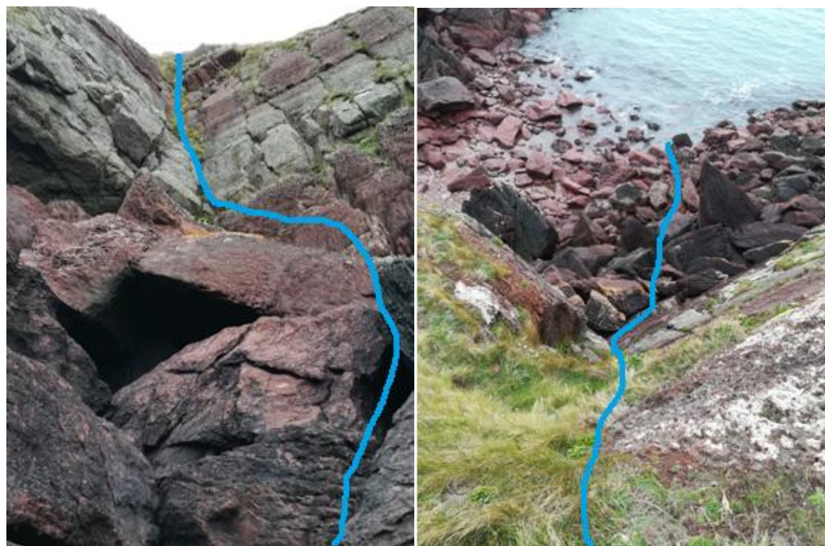
Figure 16.6 Cable route looking up and down gully
