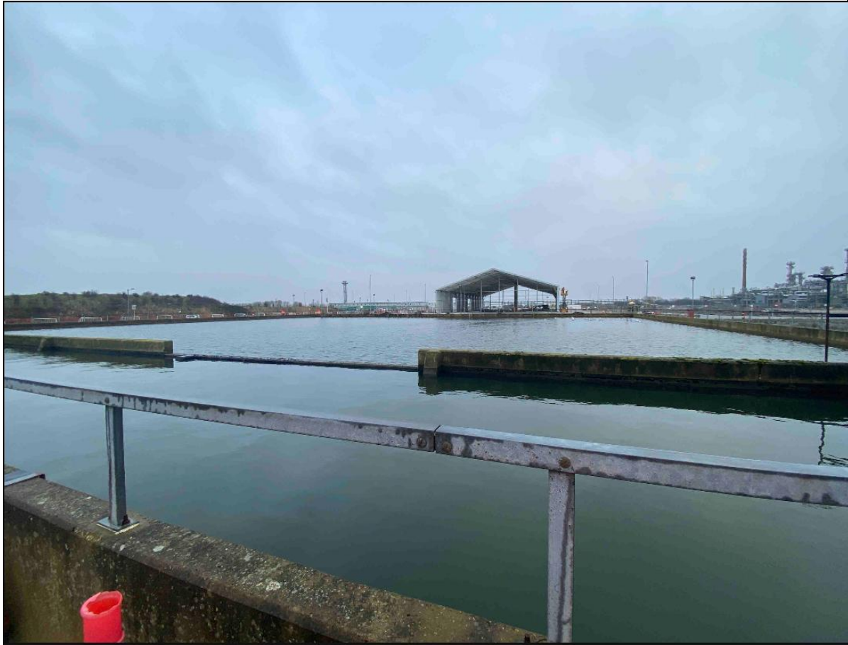
Photograph 1: Location 00: Surface water collection tank. 50.0m by 50.0m
