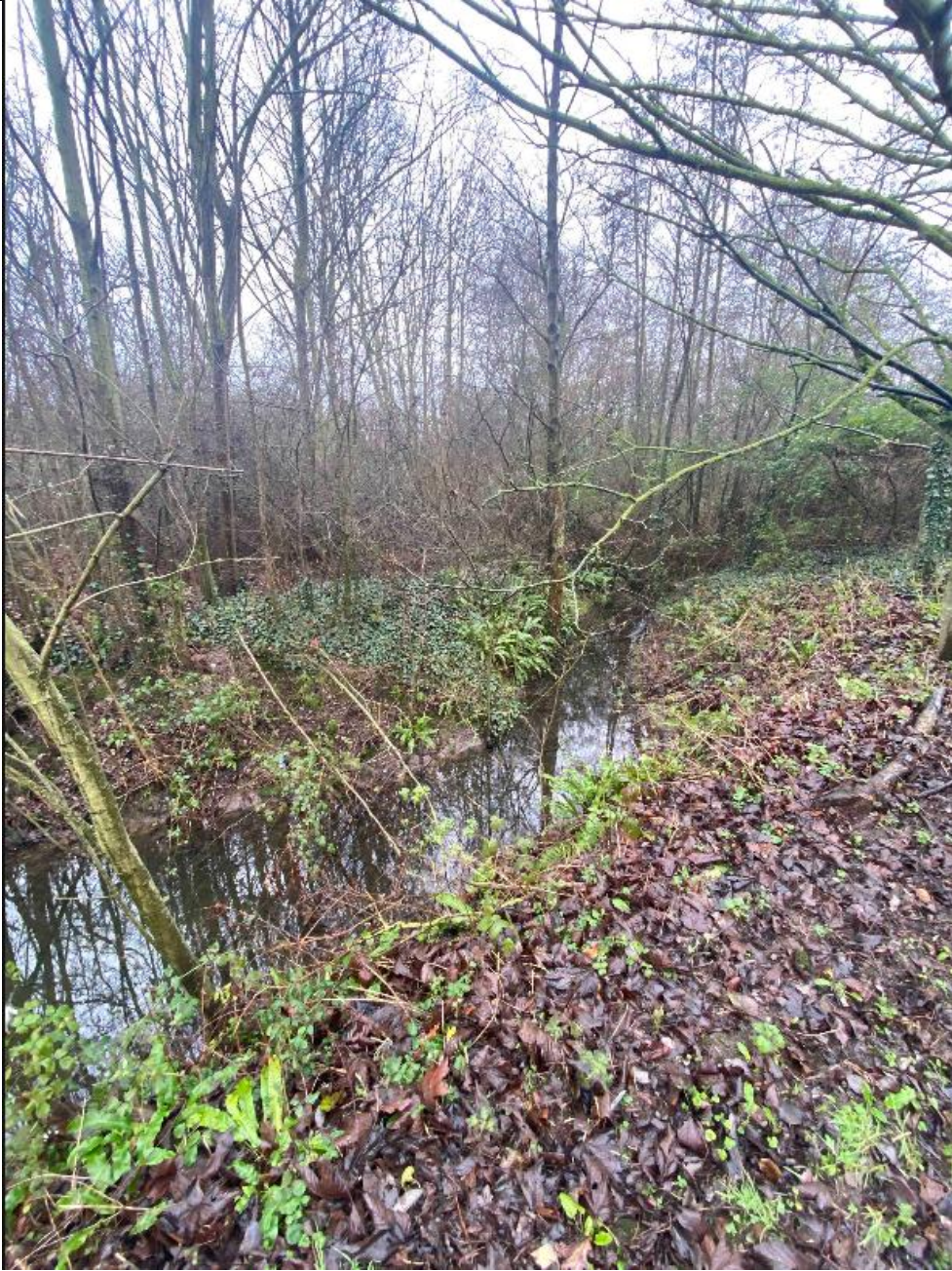
Photograph 22: Location 14: The same drainage ditch as previous location, no flow visible. Width of ~2.0m and depth of ~1.5m.
