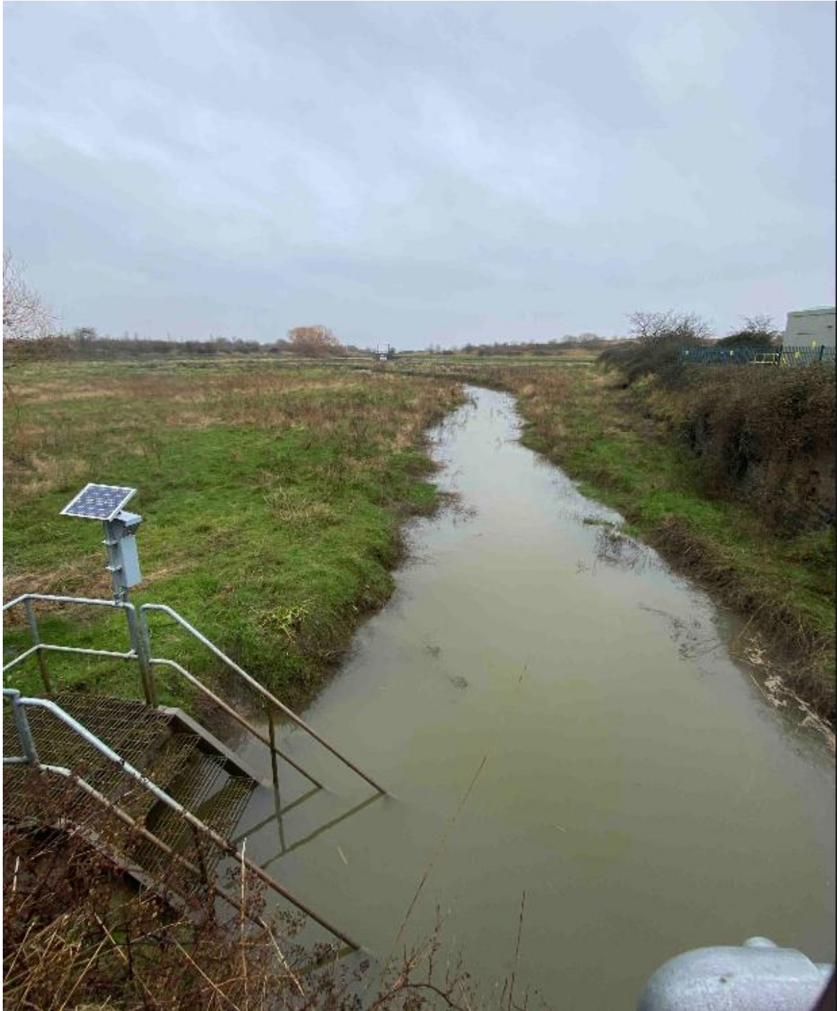
Photograph 14: Location 10: View of the outflow past the sluice gate from the lagoon. Channel is ~3.0m wide and ~1.2m deep. Photo taken facing East.
