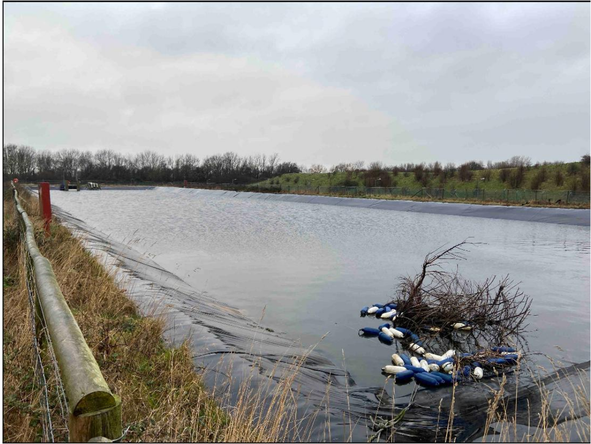
Photograph 3: Location 01: View of fire suppression water collection tank. This tank is connected to and can drain to the surface water collection tank. Currently it is cut off as it is contaminated with PFOS/PFAS. 117.0m by 30.0m
