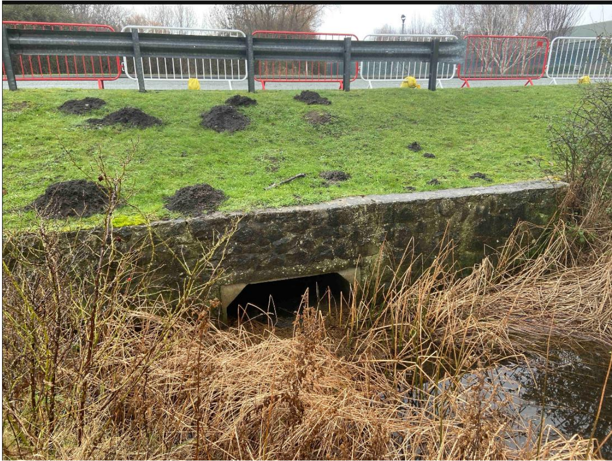
Photograph 7: Location 05: Box culvert outflow from entrance roadway for gas terminal. The culvert maintains the same shape as previous location. Box culvert is 1.4m by 0.7m and brook widens to ~6.5m wide by ~1.4m deep. No observable flow. Photo taken facing North.
