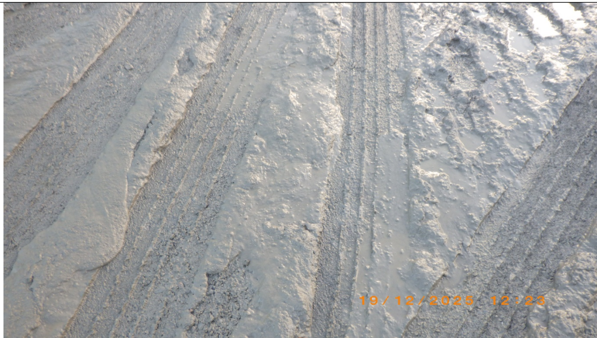
Mud on site
