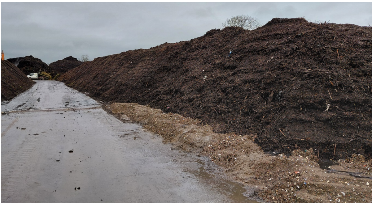
Figure 4 Photo showing concrete bump and bunding to base of longest windrow.
