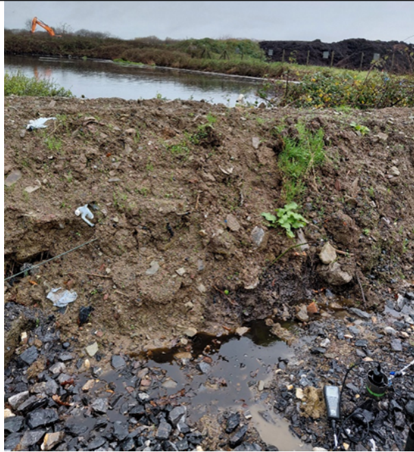
Figure 10 photo above shows high leachate level and breach of containment with dark brown/black liquid pooling outside containment.
