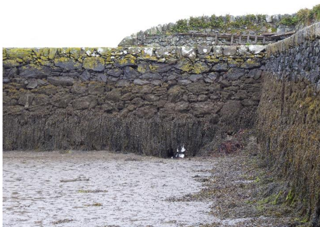
PHOTO 3.3 THE WALL AND BREAKWATER
