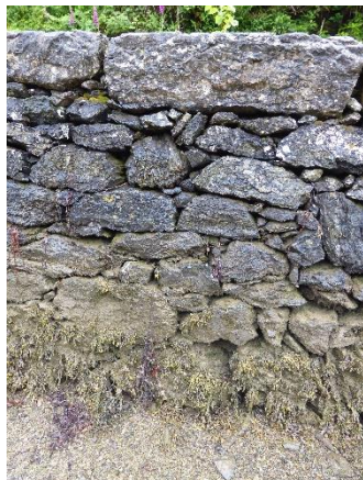
PHOTO 3.8 DETAIL OF WALL
