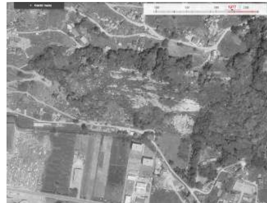
The aerial photo of 1977 shows a landslide a hundred meters from the buildings.
