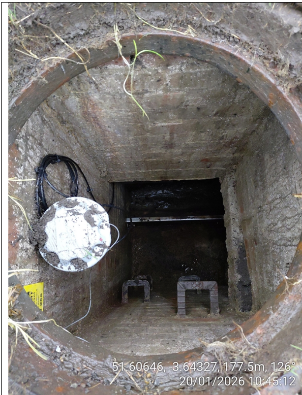
Image 1: CSO chamber to the rear of Heol y Llwyni
