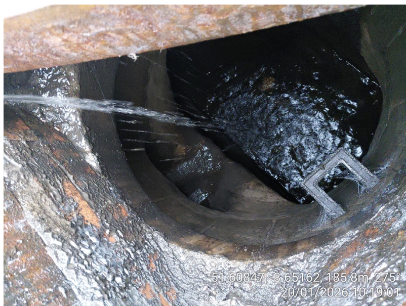
Image 2: Discharge to culvert.
