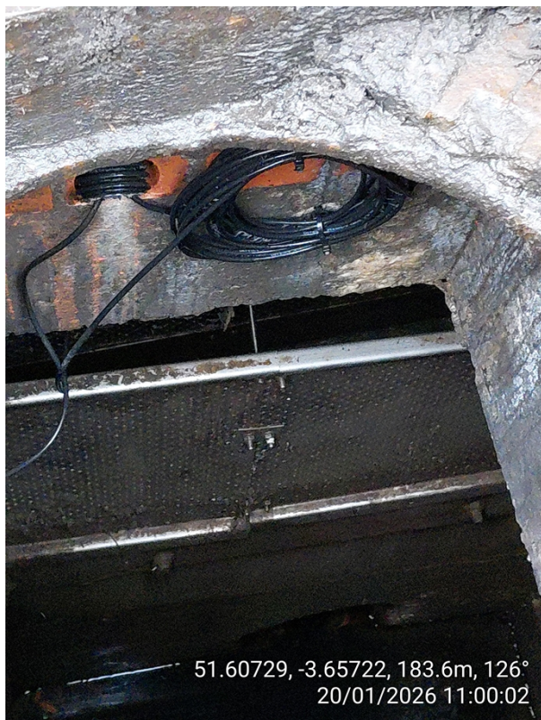
Image 2 - close up of screen in CSO chamber
