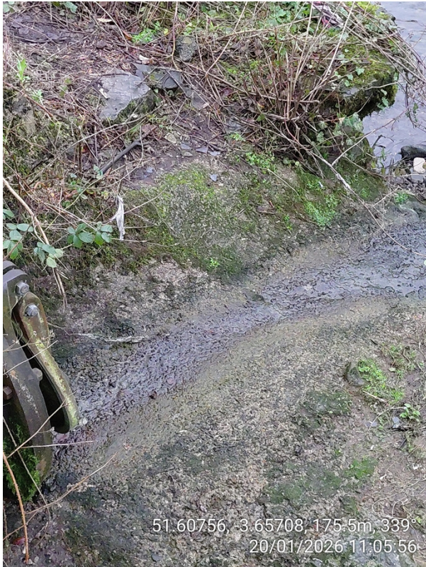
Image 3: CSO discharge location to Llynfi
