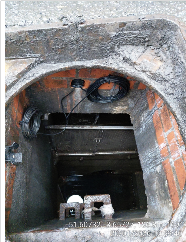
Image 1: CSO chamber on Church Street
