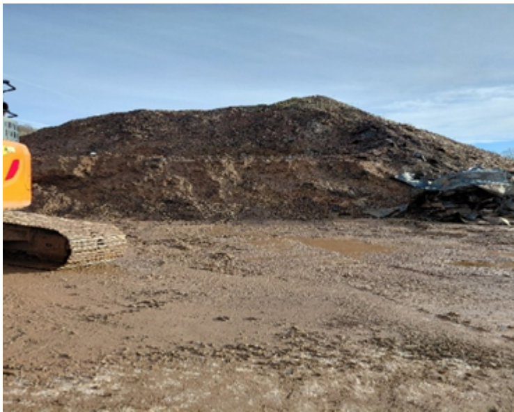
Photo 2 - shows topsoil being stored
