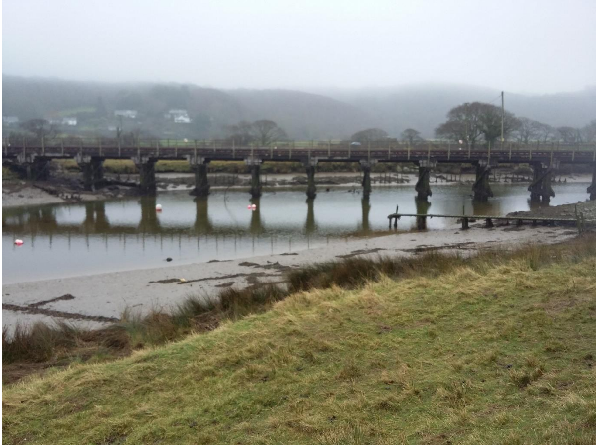
Photo of existing viaduct at low tide
