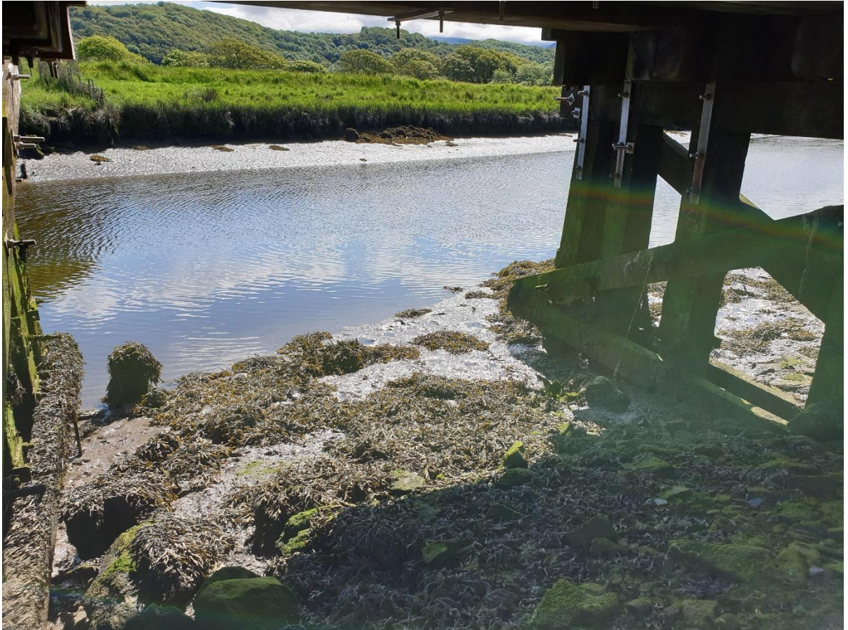
1t excavator access route picture 1 of 2
