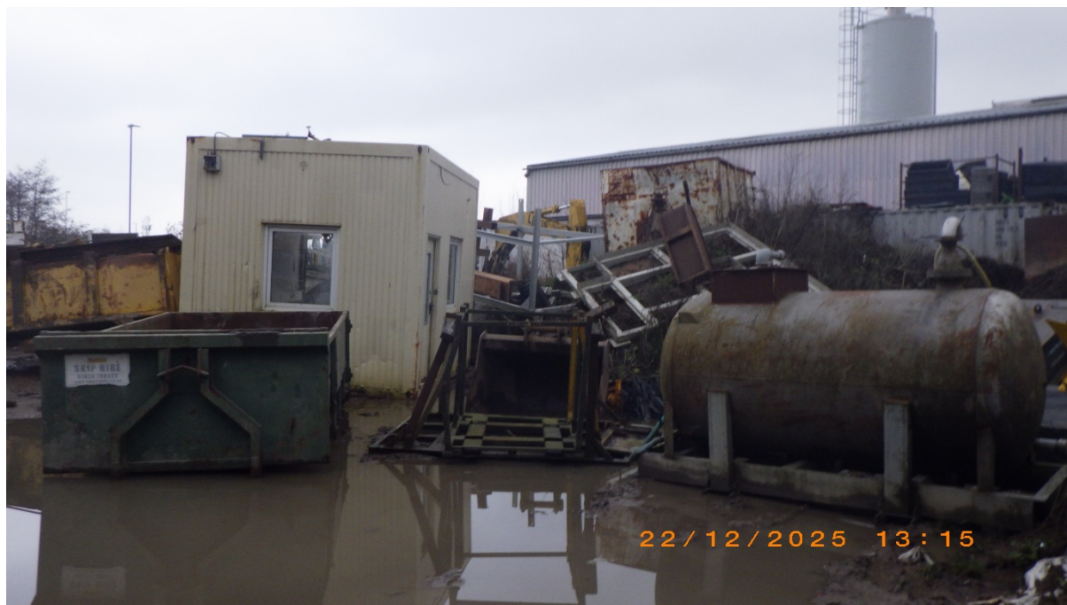
Water pooling in the yard
