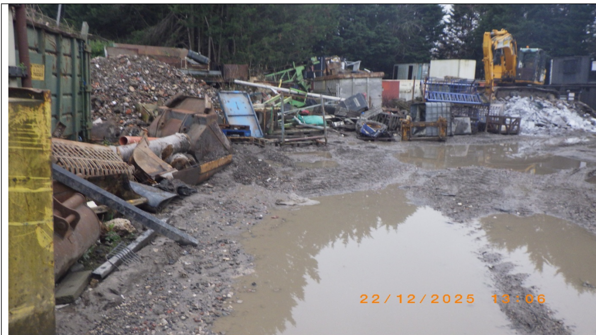
Standing water in the yard
