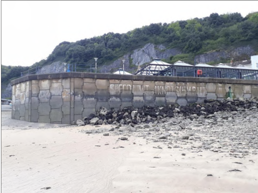
Plate 36. Sea defence wall and promenade. View to the south-southeast.
