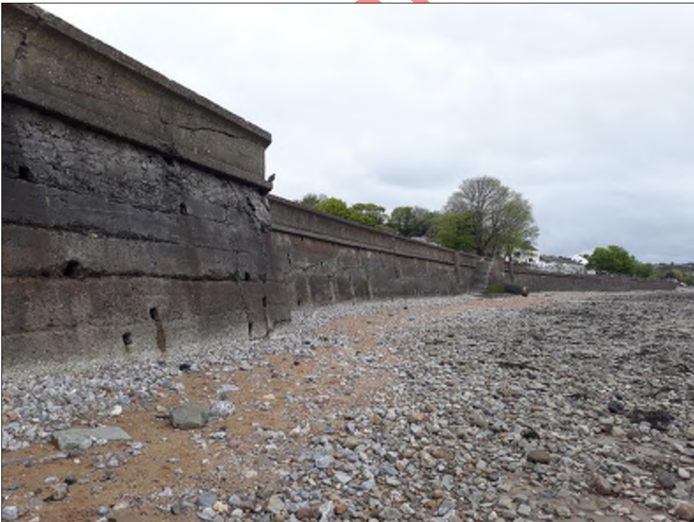
Plate 15. Sea defence wall along Oystermouth Car Park and Oyster Wharf. View to the northwest.
