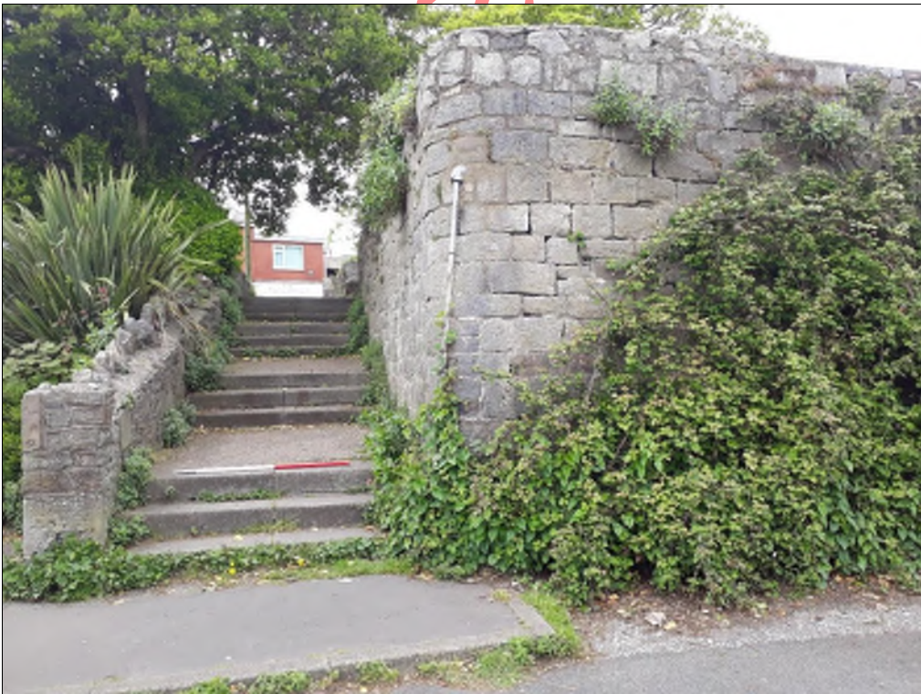
Plate 65. Steps to the upper level of Oystermouth Car Park. View to the west, scale in 0.5m divisions.
