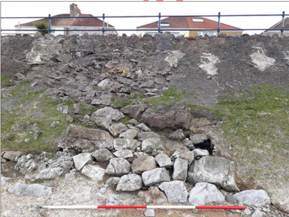
Plate 27. Detail of sea defence wall along Devon place. Note old stone wall coated with modern concrete. View to the southwest, scale in 0.5m divisions.
