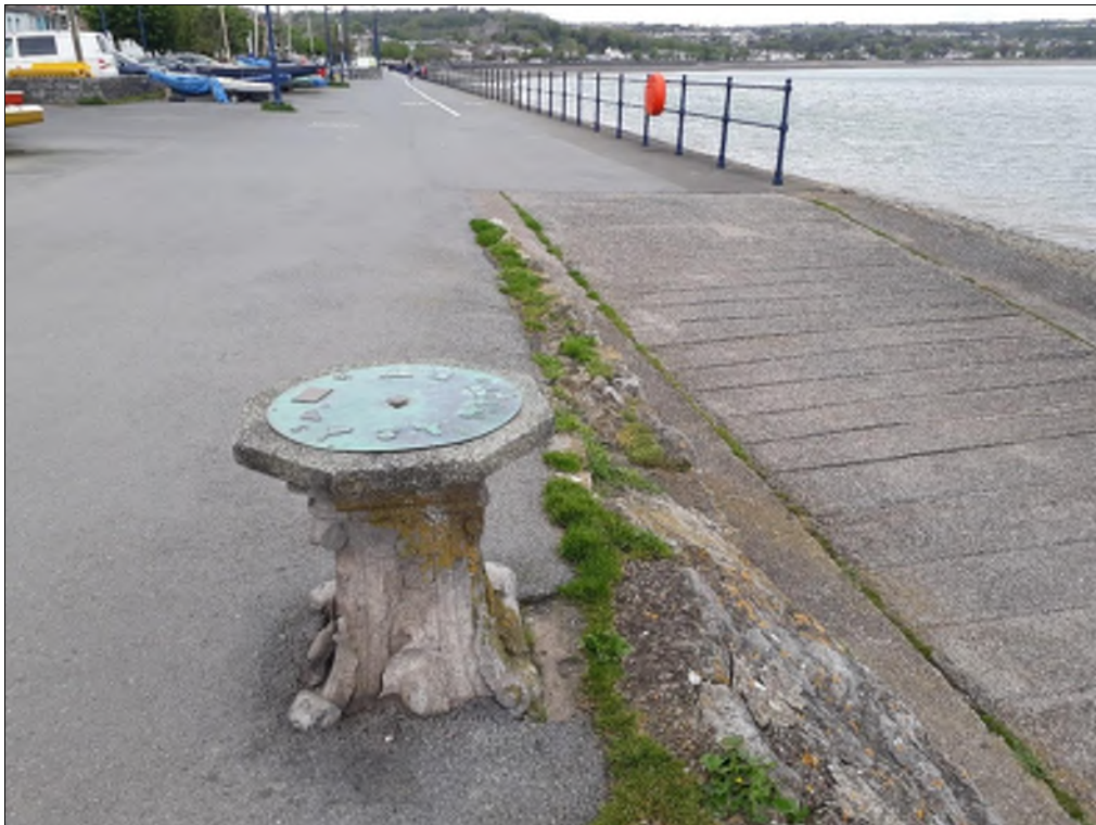
Plate 46. Promenade, edge of the slipway (05795w) and solar clock. View to the west-northwest.
