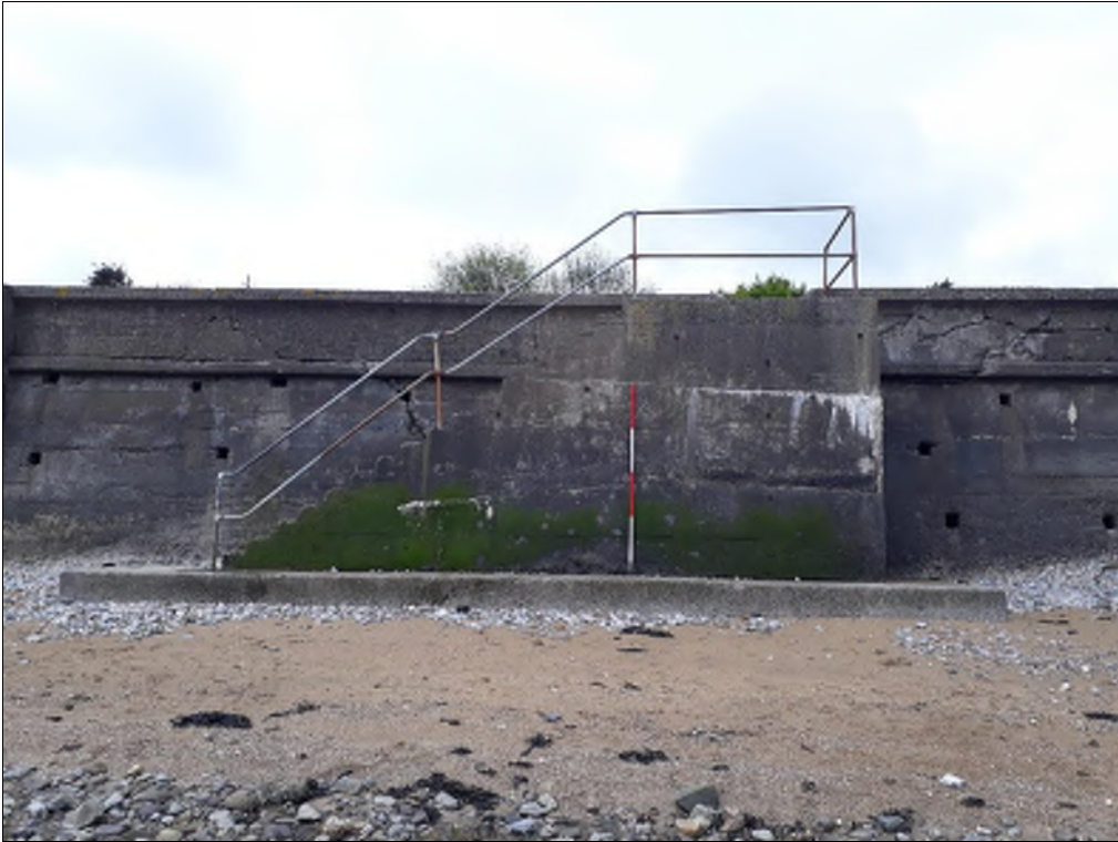
Plate 14. Detail of sea defence wall along Oystermouth Car Park. View to the west-southwest, scale in 0.5m divisions.
