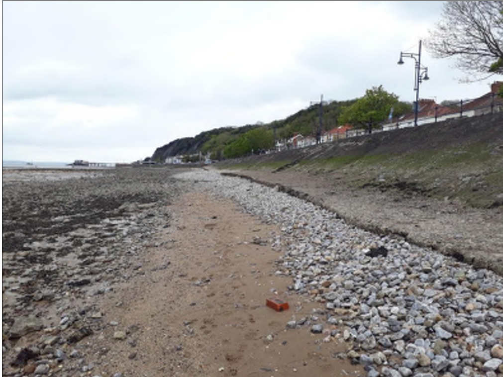
Plate 22. Sea defence wall along Devon Place. View to the southeast.
