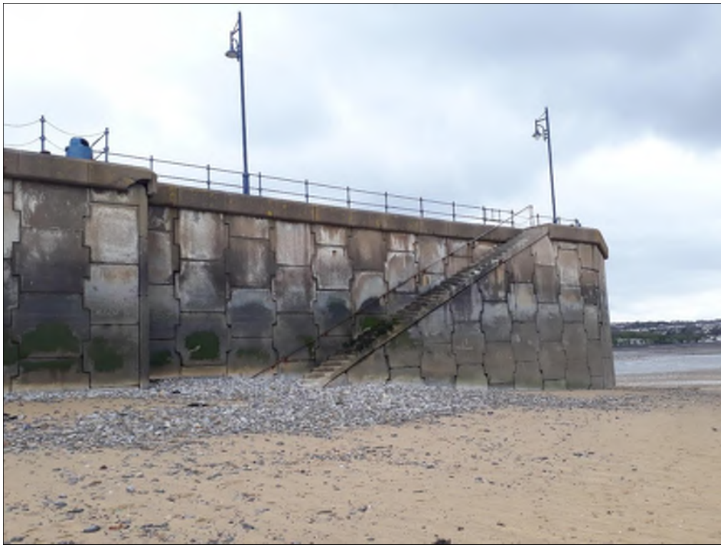
Plate 38. Sea defence wall and promenade near the Yacht Club. View to the northwest.
