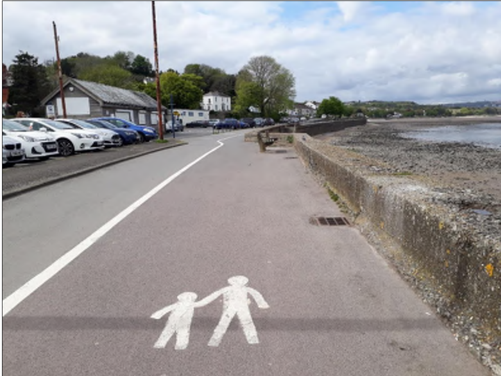
Plate 62. Promenade and carpark at Oystermouth. View to the northwest.
