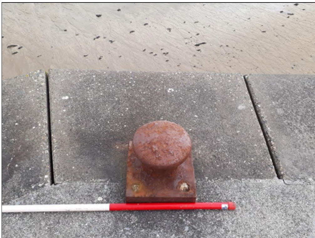
Plate 40. Mooring post. View to the northeast, scale in 0.5m divisions.
