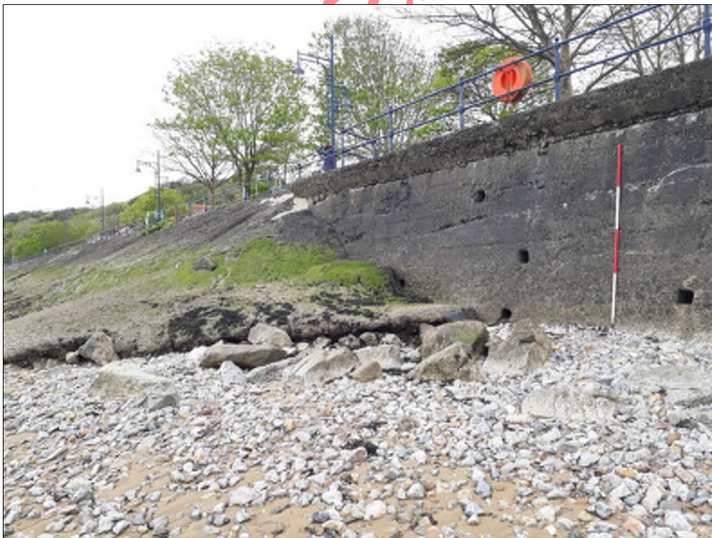
Plate 21. Sea defence wall (modern concrete wall and earlier stone wall coated by concrete). View to the south, scale in 0.5m divisions.
