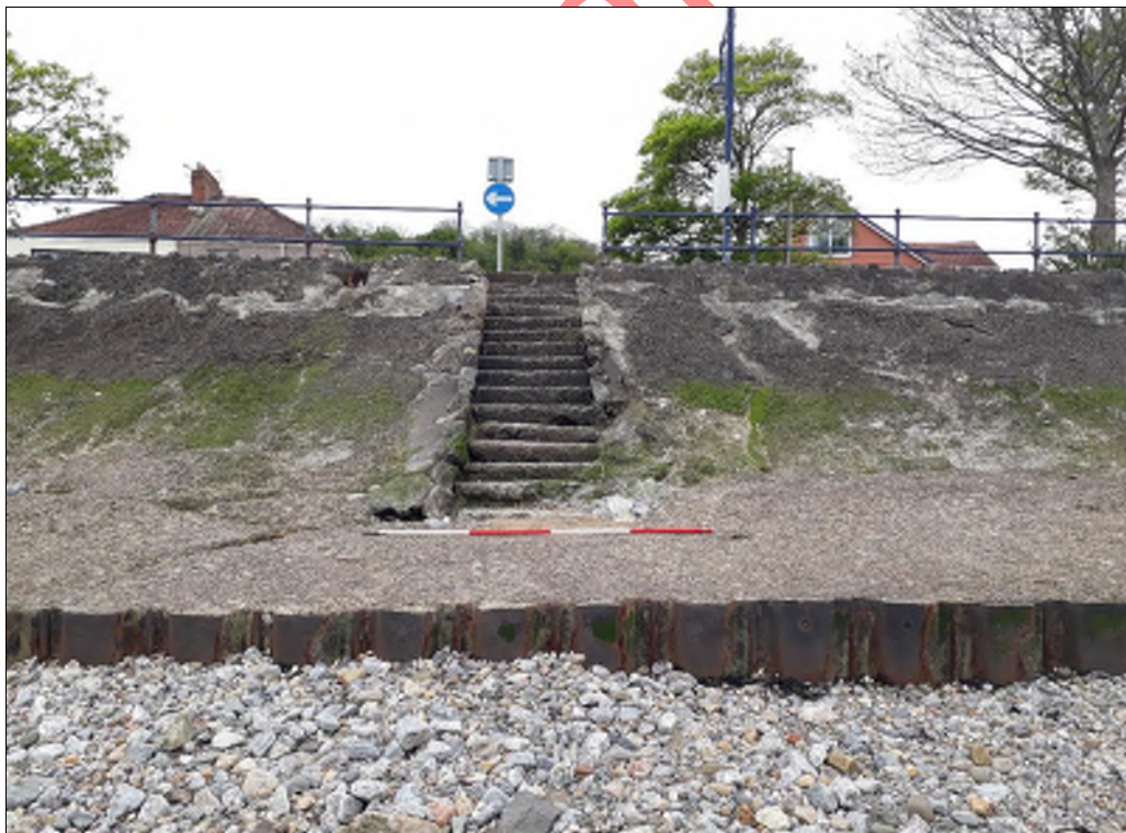
Plate 23. Sea defence wall and stairs to the front of Devon Place. View to the west southwest, scale in 0.5m divisions.
