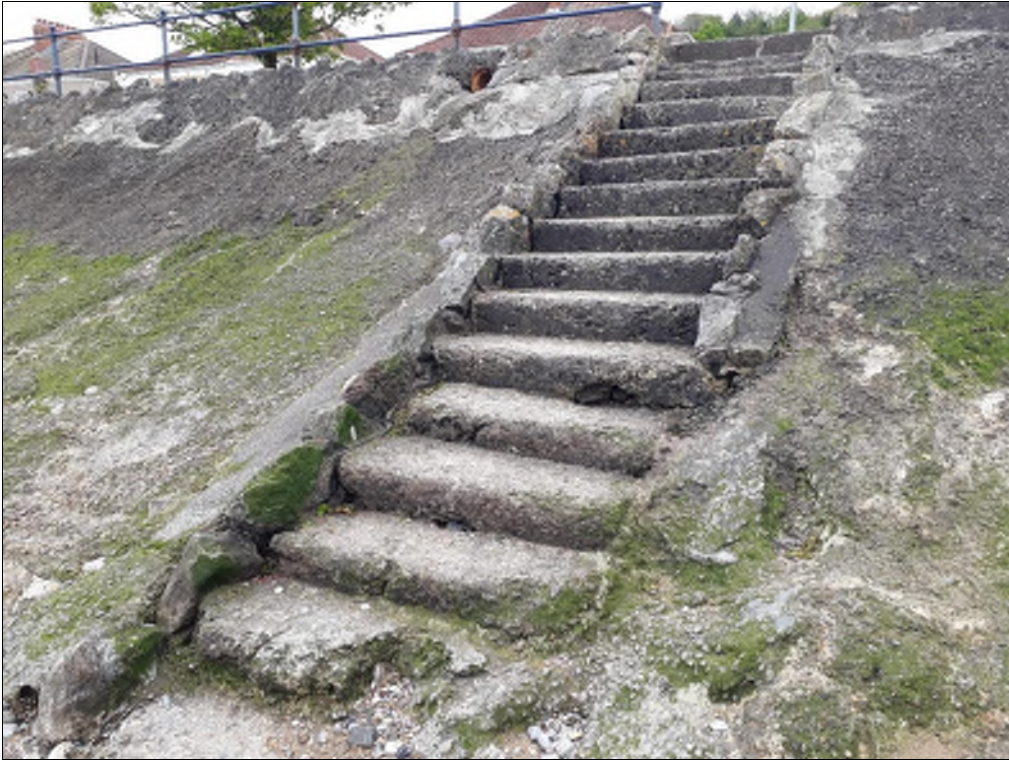
Plate 24. Detail of stairs to the front of Devon Place. Note stones used as edging. View to the west south.
