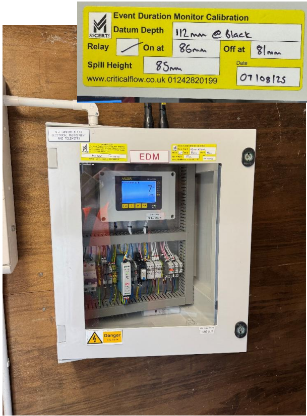
Level Meter & Label
