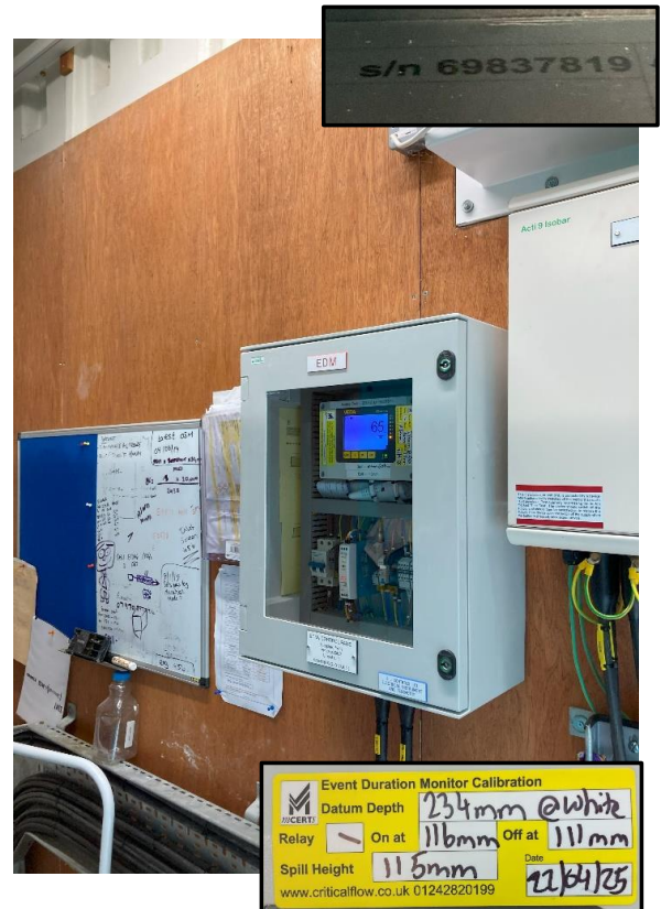
EDM Level Meter Display, Serial Number. Alarm Set Points and Datum Reference
