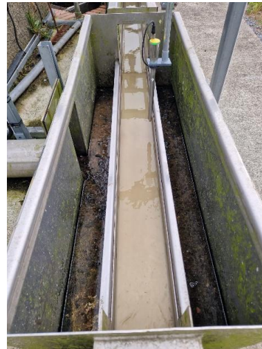
Storm Overflow Weir
