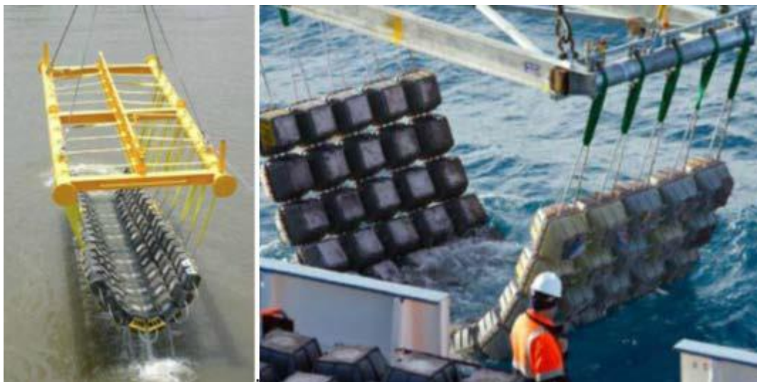
Figure 3-2 Concrete mattress deployment (courtesy of FoundOcean)
