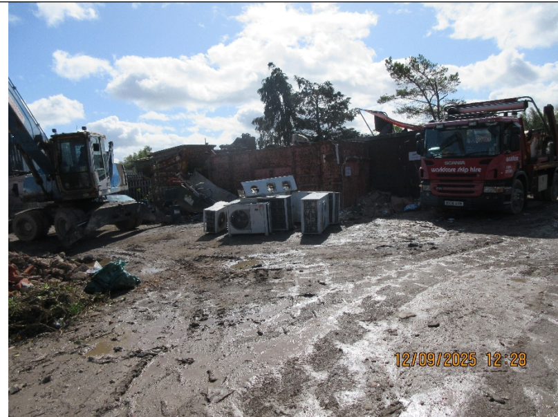
Photograph 1 - Air conditioning units stored pending removal.
