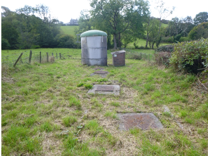
Photograph 1: Llangwyrfon STW consisting of a septic tank (foreground) and filter bed (background)
