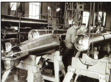
Left: G7a Torpedoes being repaired at Ostende in 1940. Top right: Model of the torpedo. Bottom right: Schematics.
