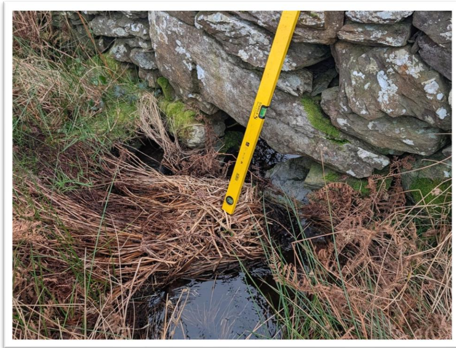
Looking downstream. Watercourse goes under wall.
