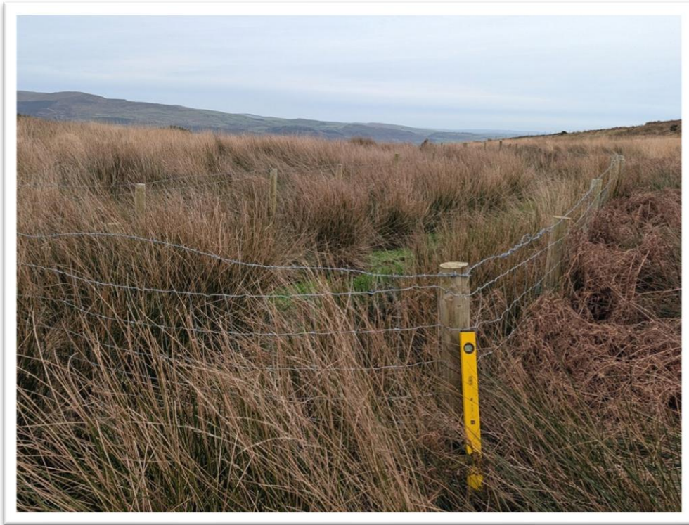
Looking downstream over impoundment towards weir.
