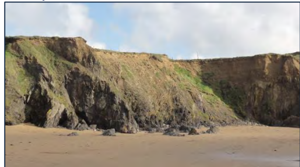
Figure 9-6: Evidence of loss of vegetation due to landslip.
