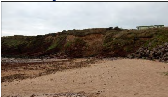
Figure 4-1: View of eroding cliffs from the rear of the cove looking east.
