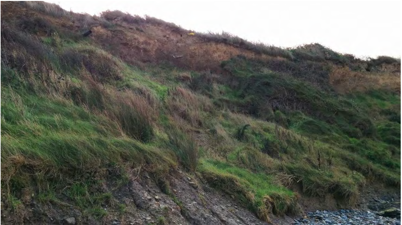
Photo 9: Soil slopes along Southern side of Boyce's Bay
