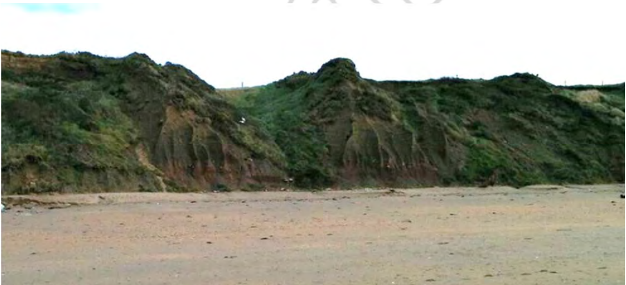
Photo 11: Slope failure along soil slopes.
