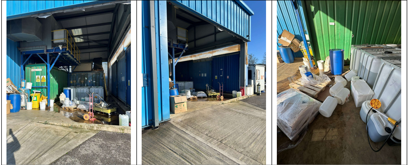
Image 1. External view of the secondary containment showing pooling of rainwater. Image 2. External view of the secondary containment showing access for forklift and/or site staff. Image 3. Empty and mixed chemical containers stored within the secondary containment.
