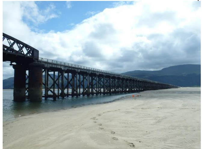
View from the north side of the viaduct
