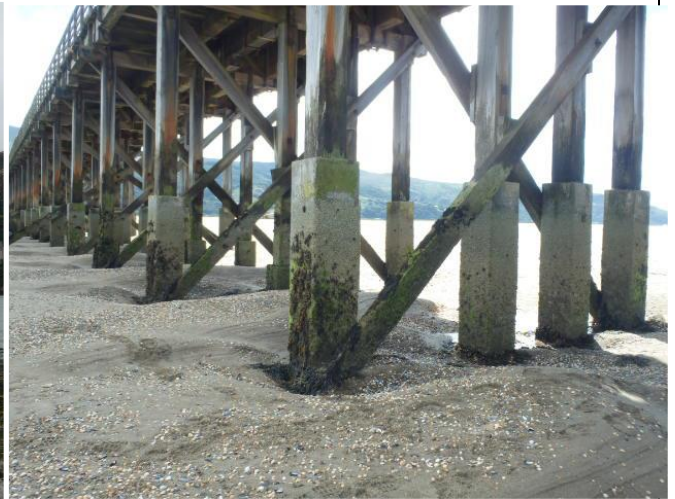
Typical works area underneath structure
