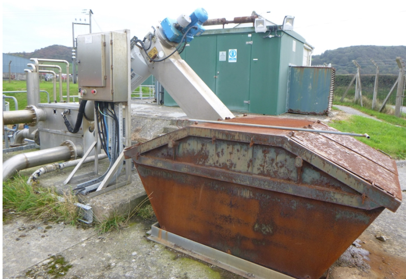
Photograph 3: Screenings deposited into skip
