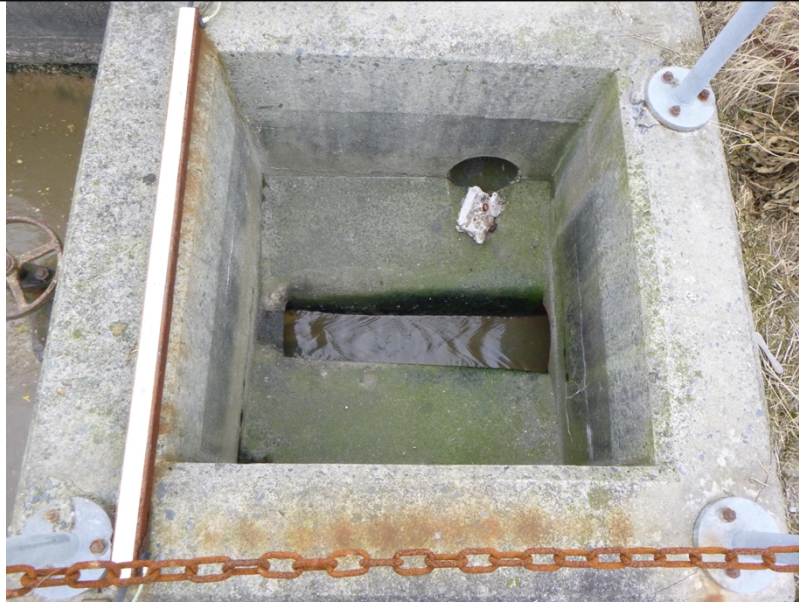
Photograph 1: Gravity inlet
