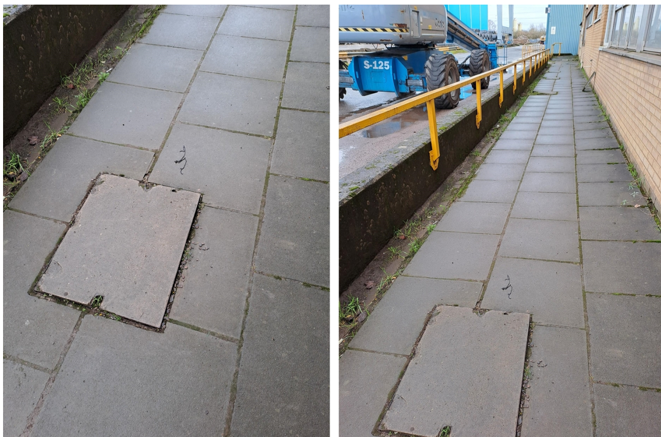
Figure 1 – Site drainage system chambers as observed during the visit.
