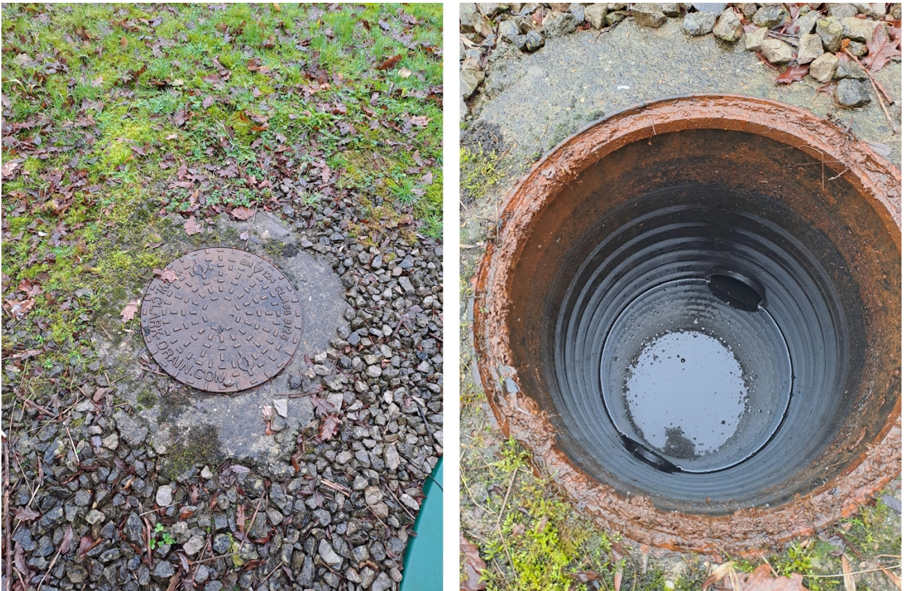
Figure 4 – The sample/discharge point chamber as observed during the visit
