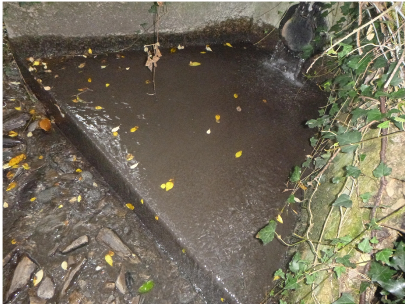
Photograph 3: Discharge point into the Nant Pant-yr-haidd
