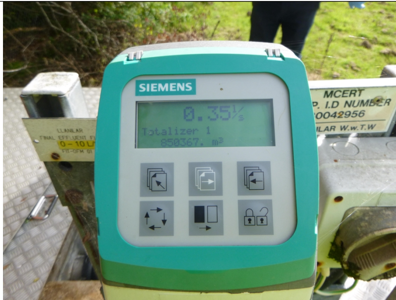
Photograph 9: MCERTS flow meter on-site visual display
