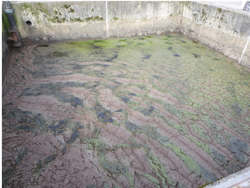
Photograph 6: Sludge holding tank
