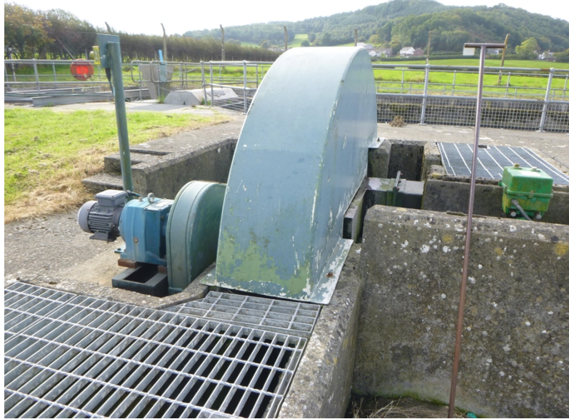
Photograph 5: Sludge lift wheel
