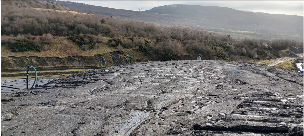
Photo 3 - Active tipping face that has not accepted waste since 05/12/25 with capping to be installed on 16/02/26 (subject to any delays). The active tipping face contains a layer of soil.
