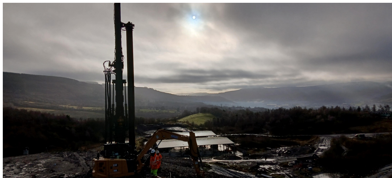
Photo 2 - Landfill gas well being installed at Bryn Pica Landfill
