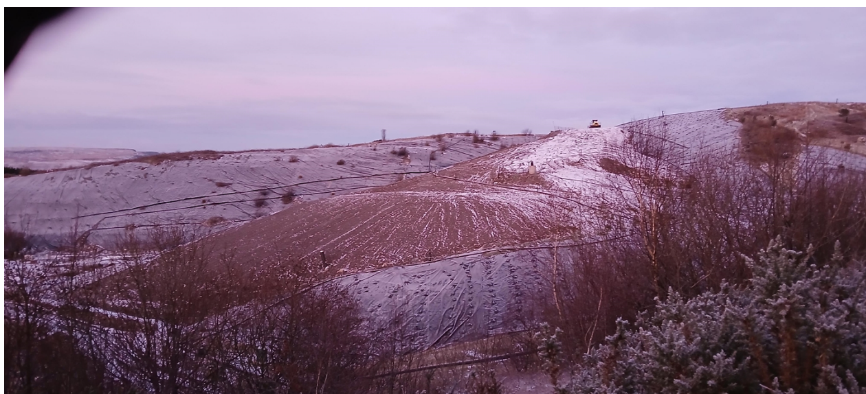
Photo 1 - Tipping face of Phase 5A, partially covered in soil and non-operational
