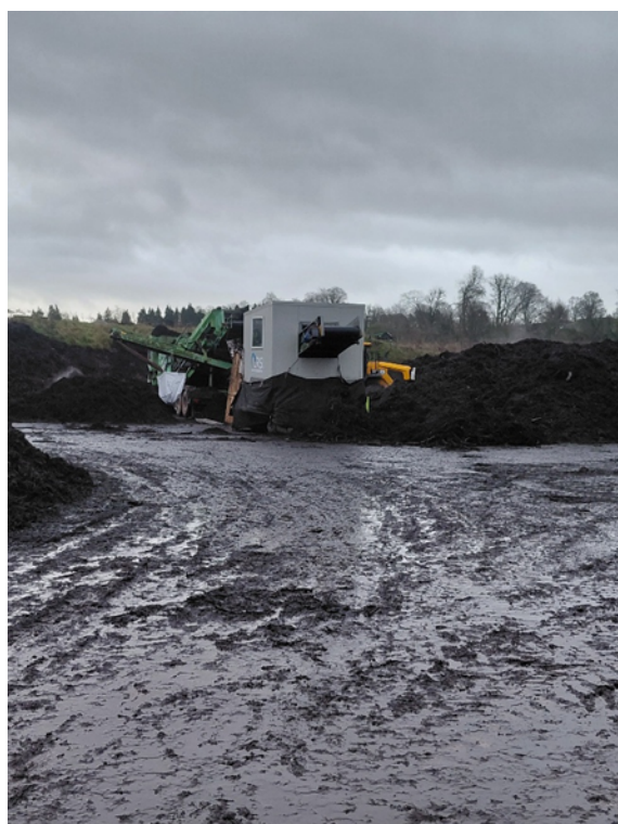
Figure 2 : Manual picking line for contaminants (Covered conveyor for all weather operation)
