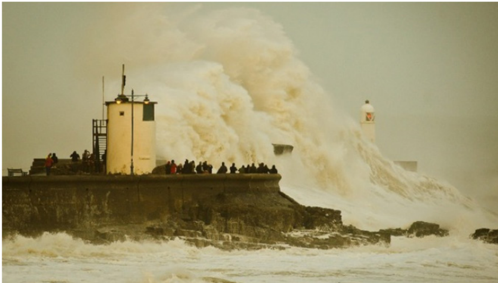
Figure 15. Wave overtopping along Porthcawl Point during a storm event on 12/02/2014
