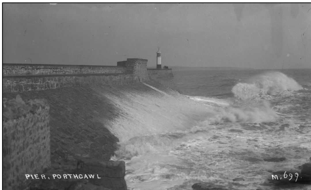
Plate 28. The Western Breakwater: glass plate negative of the Pier, Porthcawl, undated (c. 1905). 48 Courtesy of the Glamorgan Archives (GRO D261/M699).
