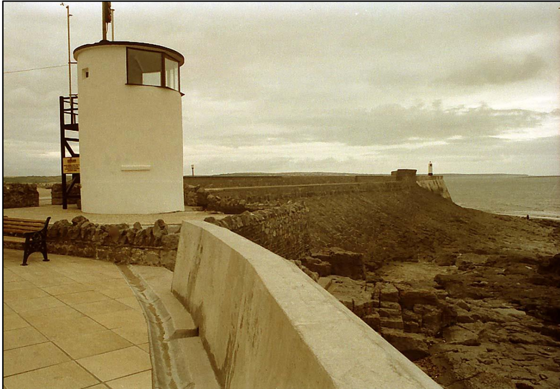
Plate 1. The Western Breakwater: view from near the Look-out tower towards the light house
