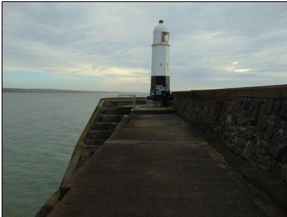
Plate 9. The Western Breakwater: the lighthouse and steps at the round end.
