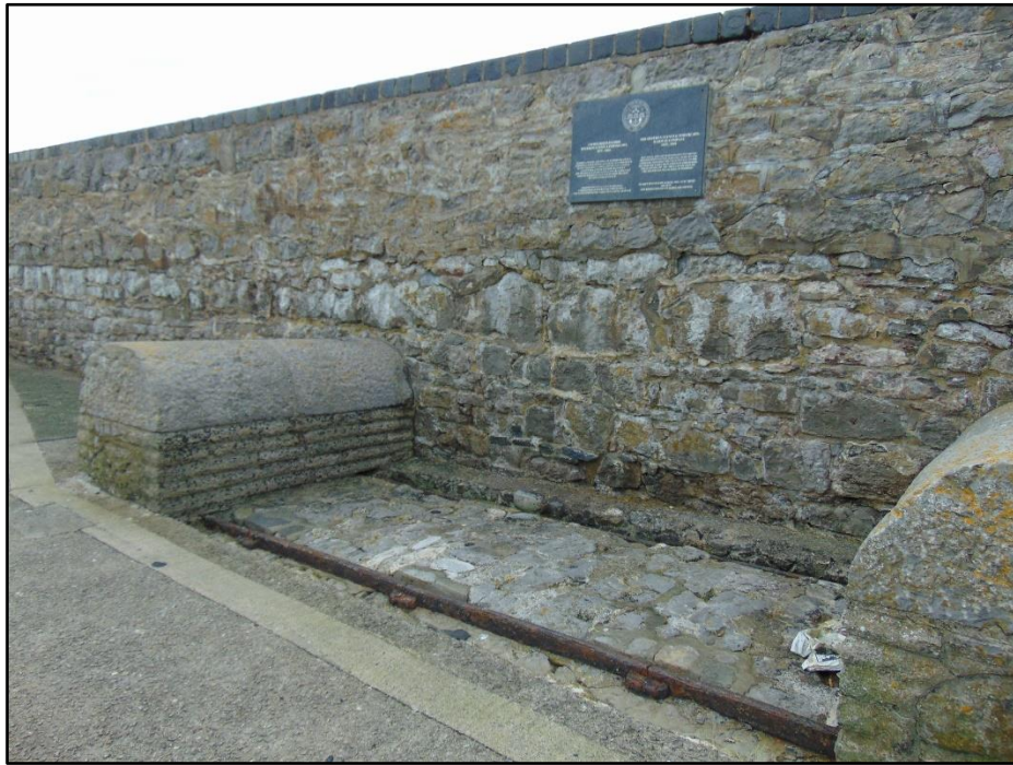
Plate 6. Western Breakwater: section of Dyffryn Llynfi Porthcawl Railway and upper wall.
