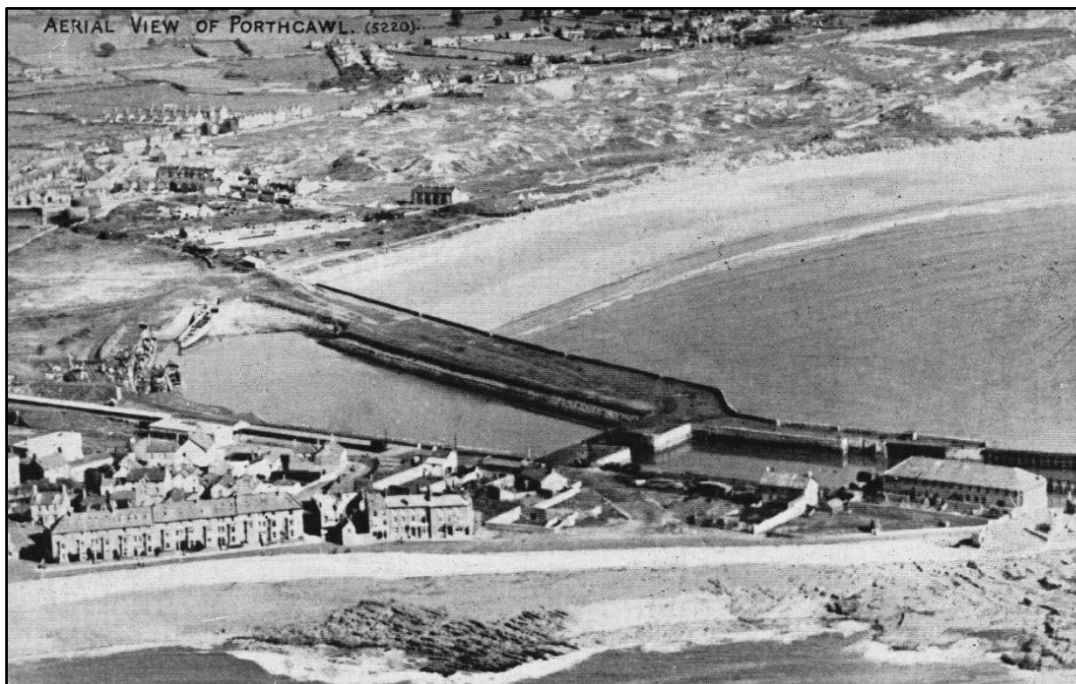
Plate 38. Porthcawl Docks: aerial Photograph, 1919-1926. Courtesy of Porthcawl Museum.
