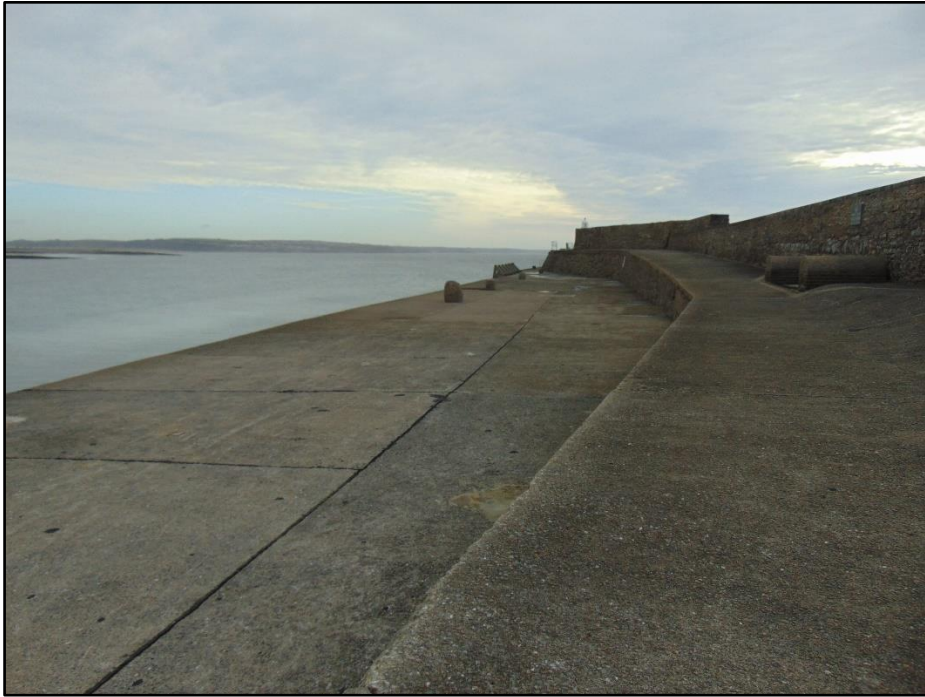
Plate 5. The Western Breakwater: the quay (steamer berth) and the section of railway from above. Taken from near the Customs House.
