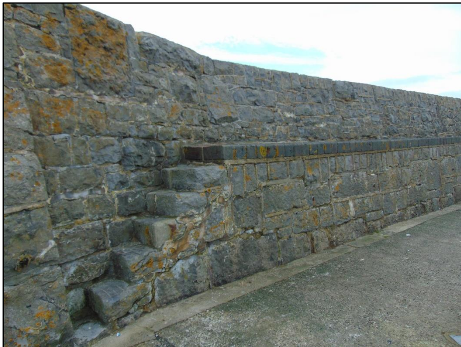
Plate 7. The Western Breakwater: steps and upper wall, inner side of junction with the extended section of the 1860s.
