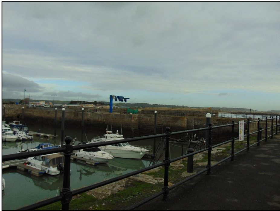
Plate 13. The Outer Basin: the east wall
