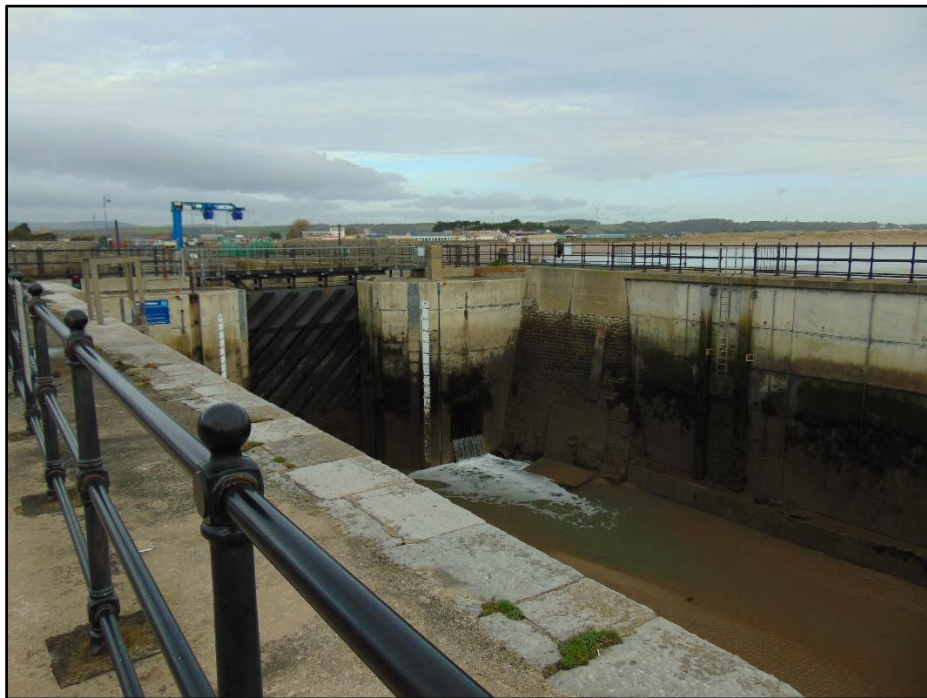
Plate 14. The Outer Basin: entrance gates to the marina
