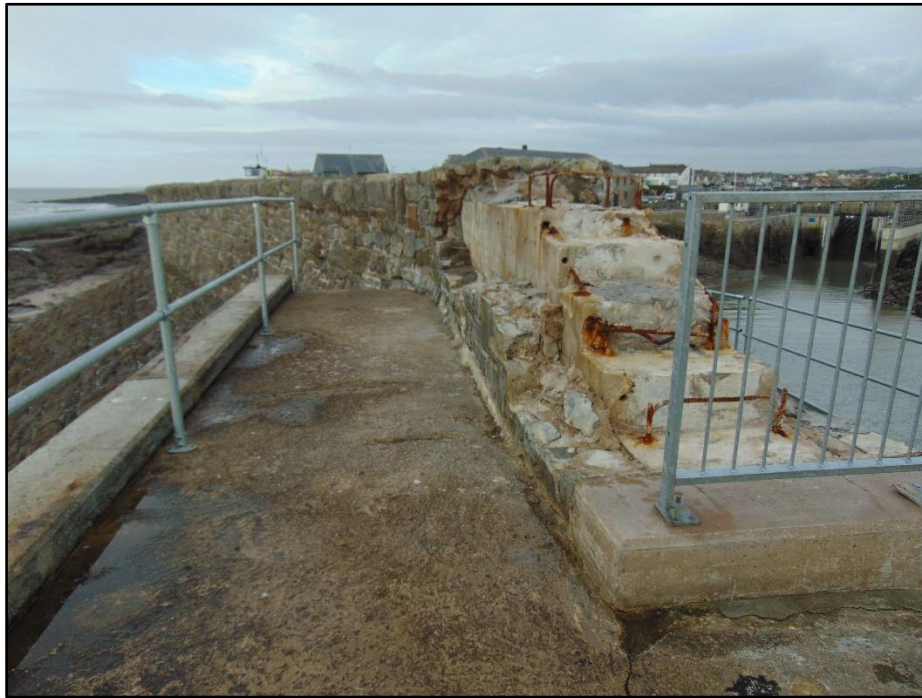
Plate 8. The Western Breakwater: the junction between the extended section of the 1860s (foreground) and the original part of the breakwater.
