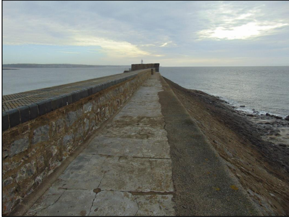
Plate 10. The Western Breakwater: wall and walkway on seaward side with sloping revetment below to the right. Taken from south of the Lookout Tower.
