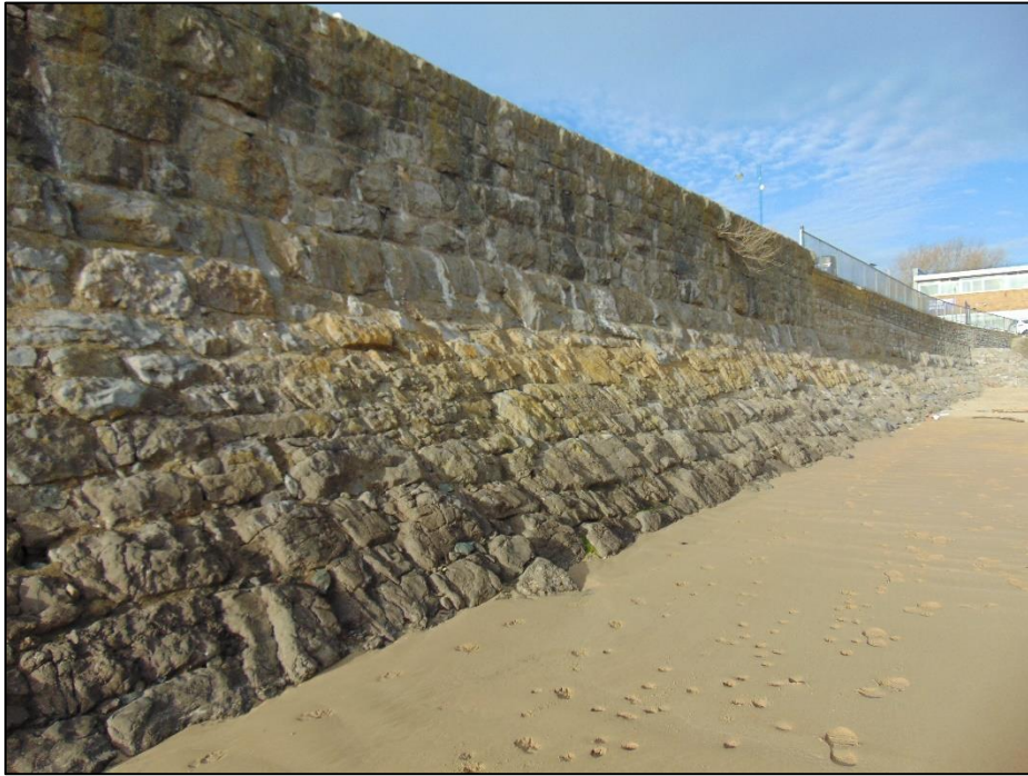
Plate 19. Eastern Promenade: Inner Basin/promenade wall and revetment towards the Coney Beach end
