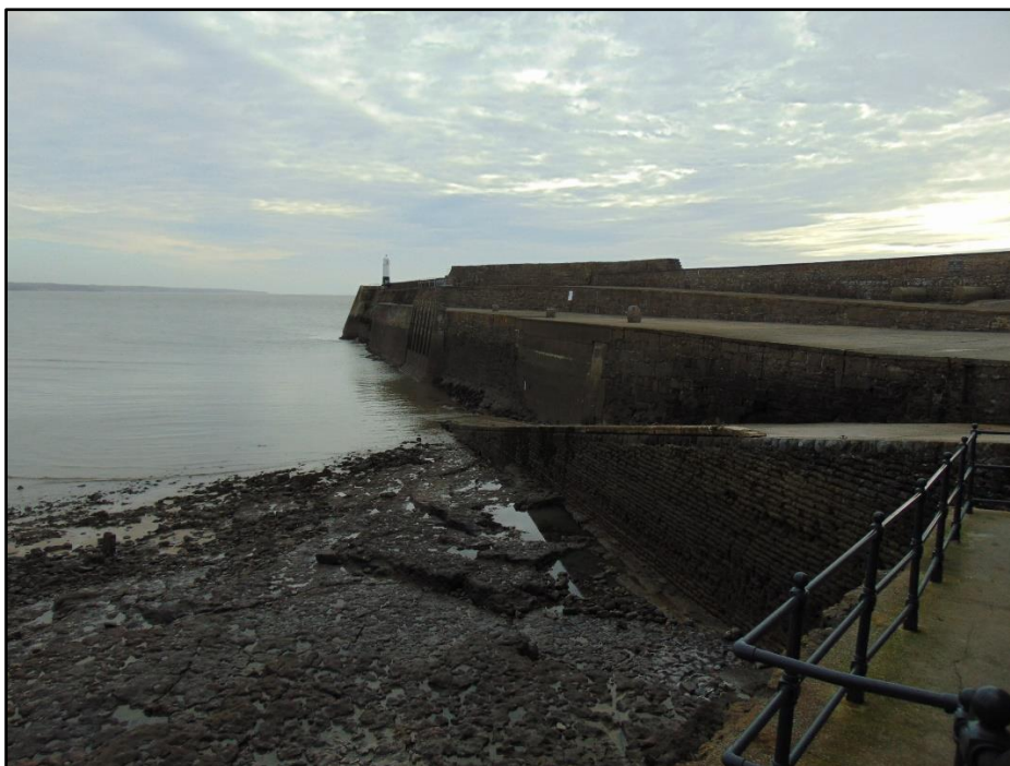
Plate 3. The Western Breakwater: tiered layout on the landward side and adjacent slipway. Taken from West Quay and Jennings Warehouse.
