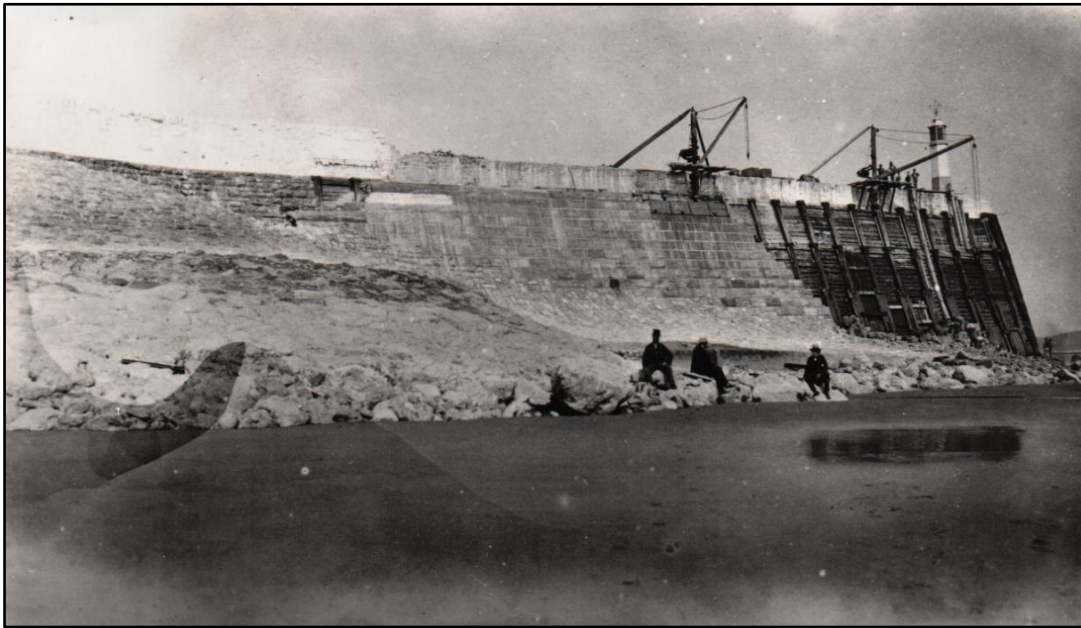
Plate 25. The Western Breakwater during later stages of construction: photograph of c. 1866. Courtesy of Porthcawl Museum.
