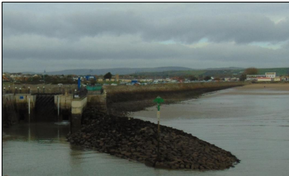
Plate 16. Eastern Promenade: view of Outer Basin (left) with Inner Basin Wall extending to Coney Beach (right)
