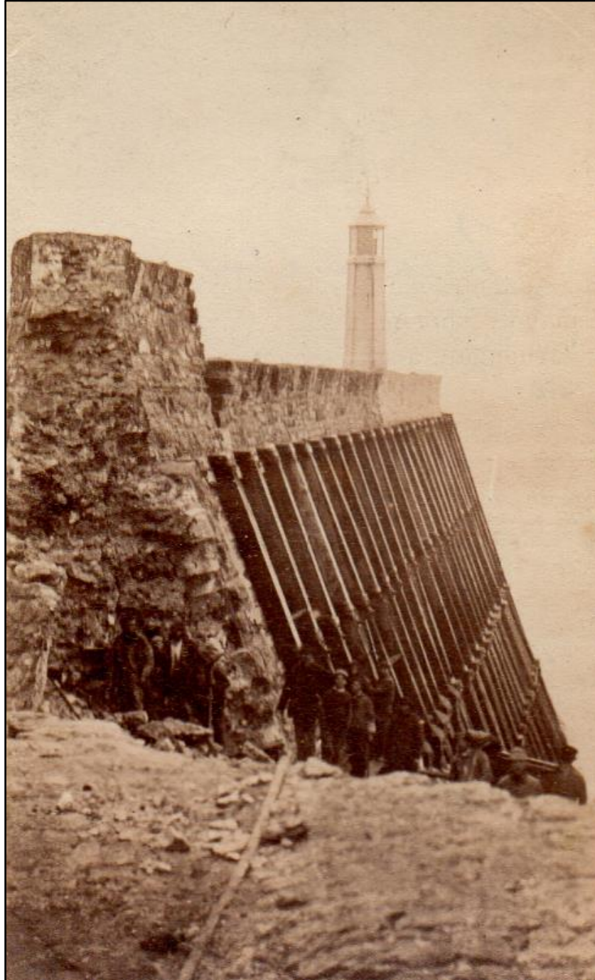
Plate 24. The Western Breakwater during later stages of construction: photograph of c. 1866. Courtesy of Porthcawl Museum.
