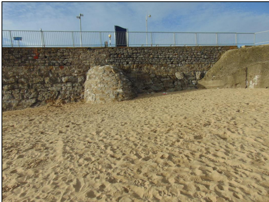
Plate 20. Eastern Promenade: Inner Basin/promenade wall and revetment at the lower Coney Beach end
