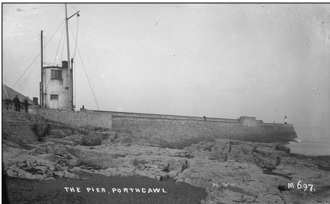
Plate 26. The Western Breakwater: glass plate negative of the Pier, Porthcawl, undated (c. 1905). 46 Courtesy of the Glamorgan Archives (GRO D261/M697).
