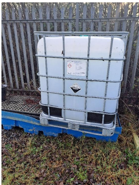
Images 1 & 2 – IBCs with lack of appropriate containment.
