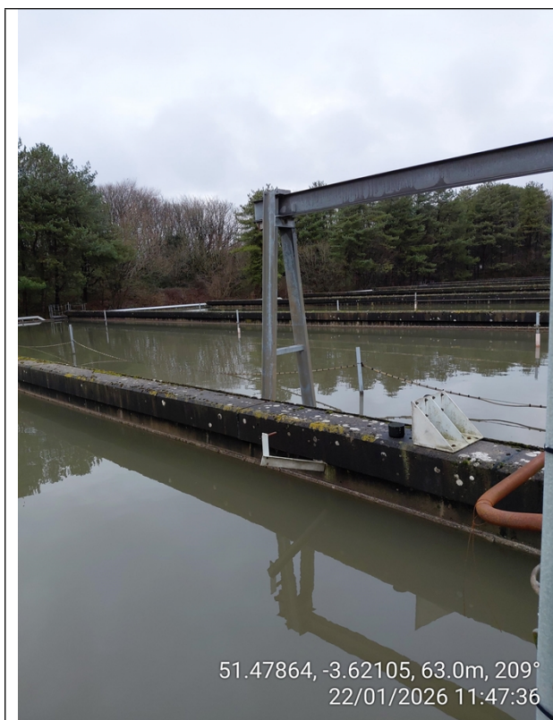
Image 2: Storm tanks (2 of 8)
