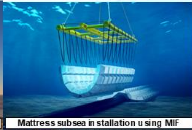
Mattress subsea installation using MIF
