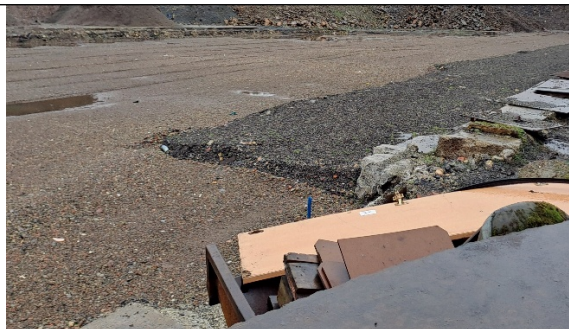
Image 4 shows on going improvement to ground resurfacing.
