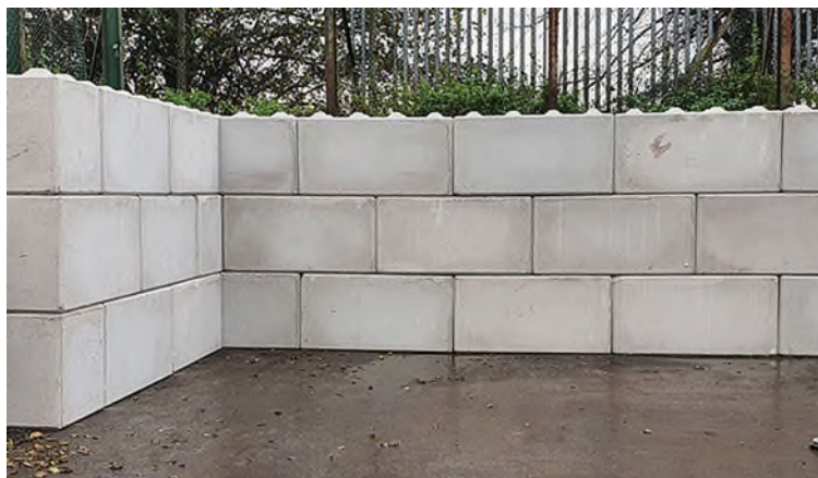
Figure 2 – Legato Block Wall Bay
