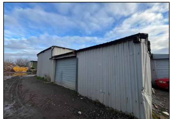
Figure 13: Example of Structures On Site.
