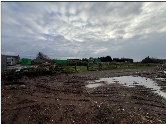
Figure 9: Bare Ground Proposed for Concreting.
